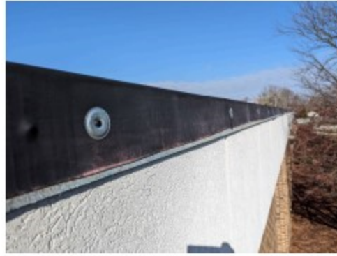
EPDM fastened to the cleat
