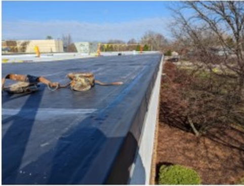
EPDM ran up and over the edge
