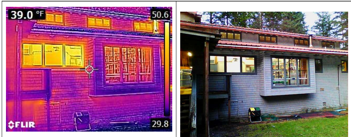
1. Windows in elementary school in reasonably good condition
