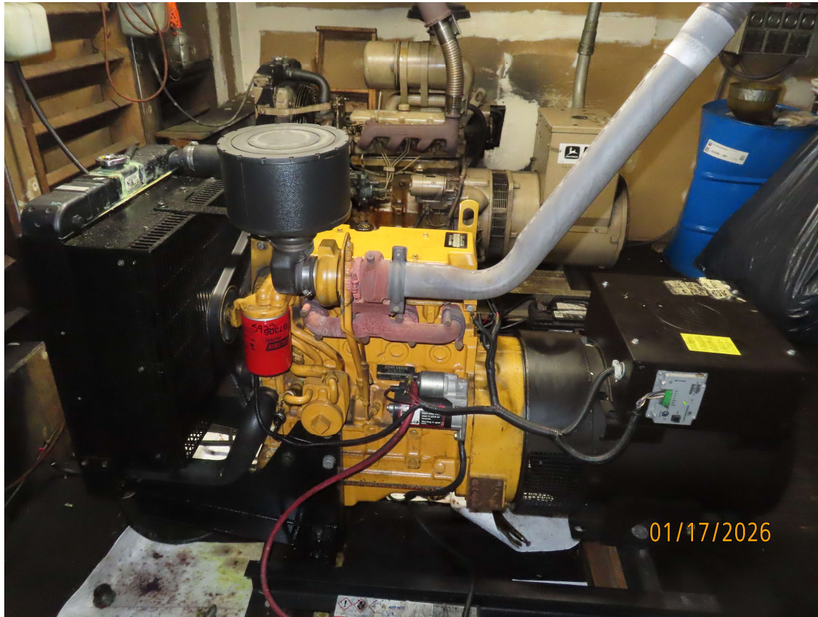
Two generators shown, only one is functional
