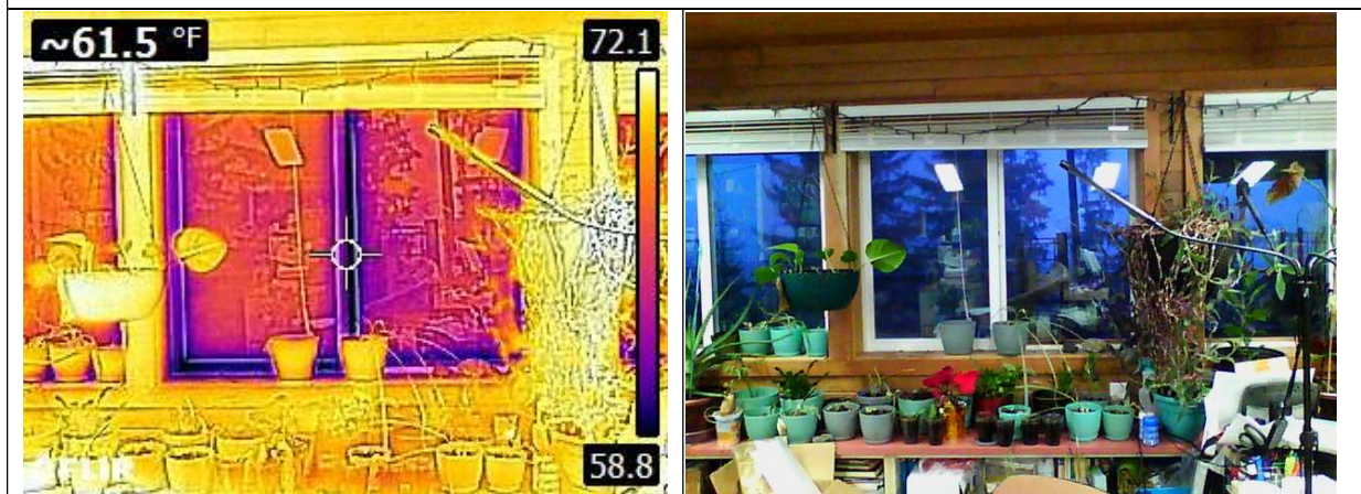
4. Windows are in good condition
