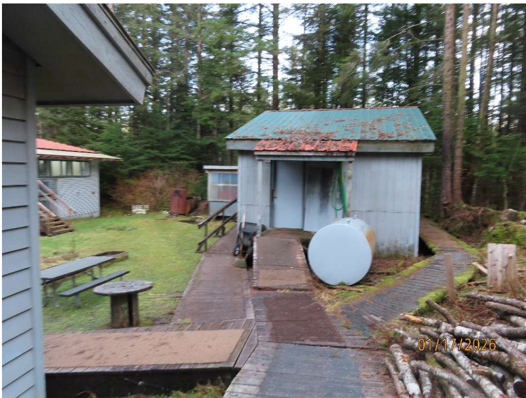
Generator shed adjacent to the school building
