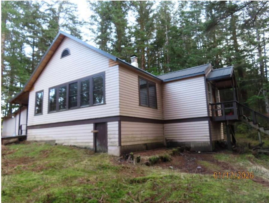
Bear Hall adjacent to the school, may share the generator output
