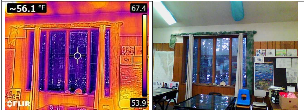
2. South windows in high school in reasonably good condition
