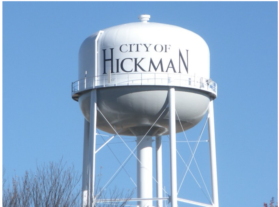
Photo 6.1: City water tower Source: Marvin Planning Consultants
