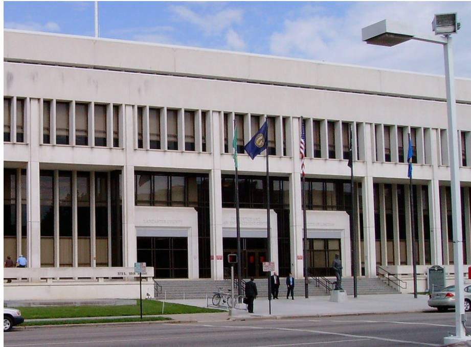
Photo 7.1: Lancaster County Courthouse - Sheriff Department's home Source: Flickr
