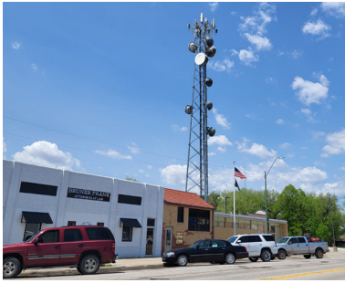
Ainsworth Cell Tower
