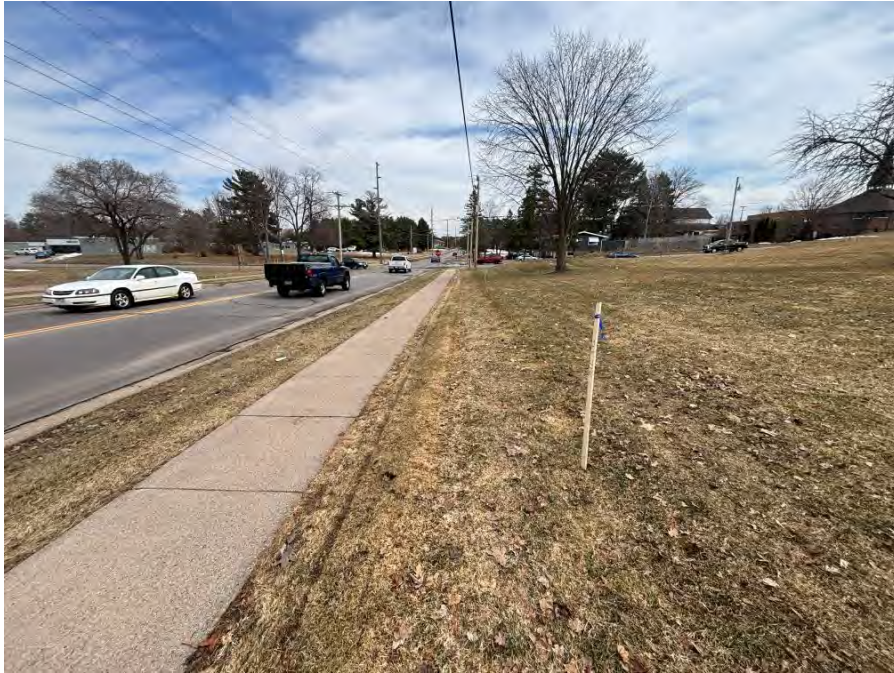
The TLE area found along Jelinek Ave in the north central part of the subject. Jelinek Ave is on the left side of the photo.
