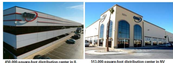
450,000-square-foot distribution center in IL
