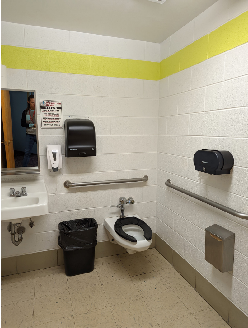
EXISTING STAFF TOILET
