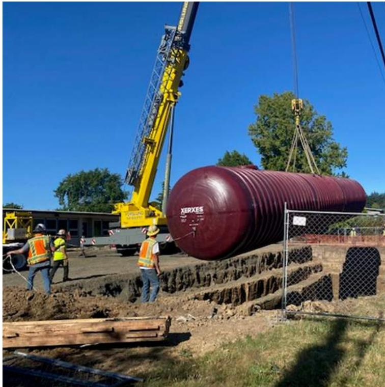
***A 40,000 gallon fire water storage tank is placed at Mt. View!***
