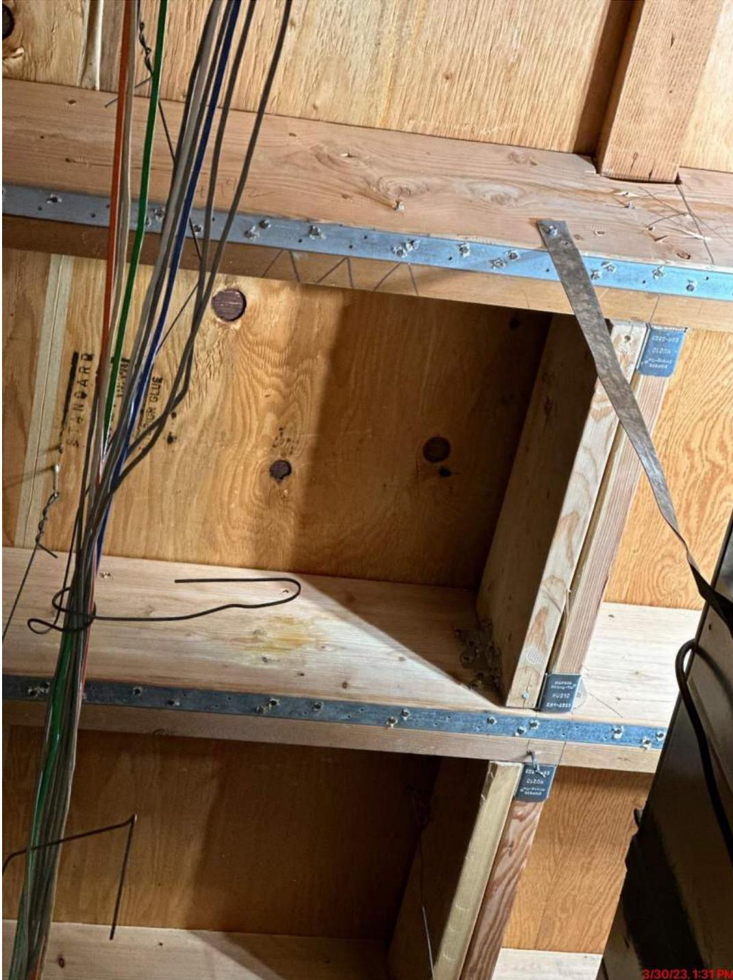
*Cheldelin – Duct penetration reinforcement*
