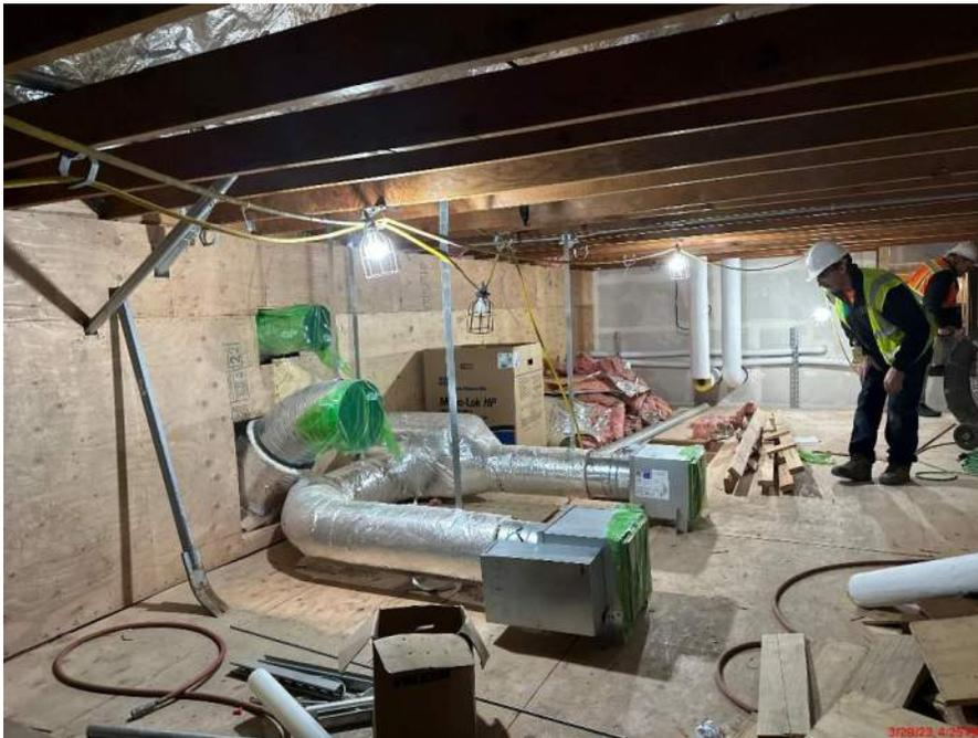
*CHHS – misc. ductwork installation in attic space*
