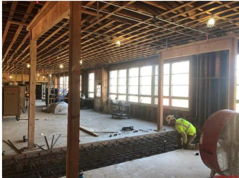
*CHHS- Shear wall footing missing from original build – added new footing*
