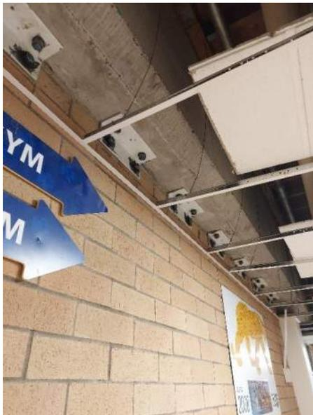
*CMS – New seismic angles in gym corridor*
