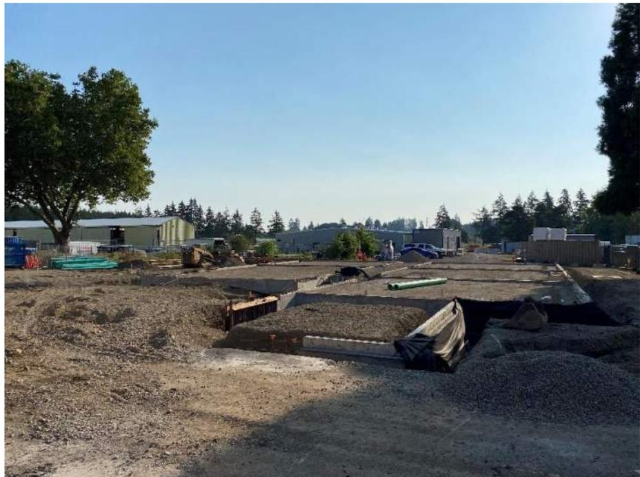
*Addition ready for concrete slab*
