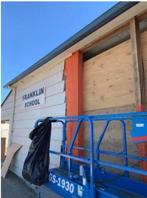
*Windows removed and waterproofing installation*
