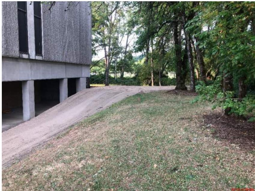
*Bldg. A – Crane Ramp for structural work (will be removed in August)*
