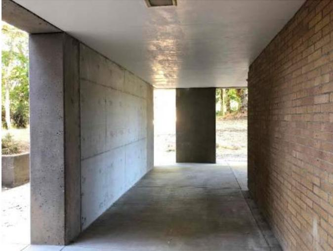
*CVHS Building A – New shear wall section and soffit repair*
