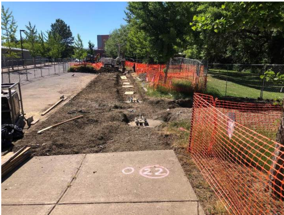
CHS – Covered Walkway piles installed or drilled
