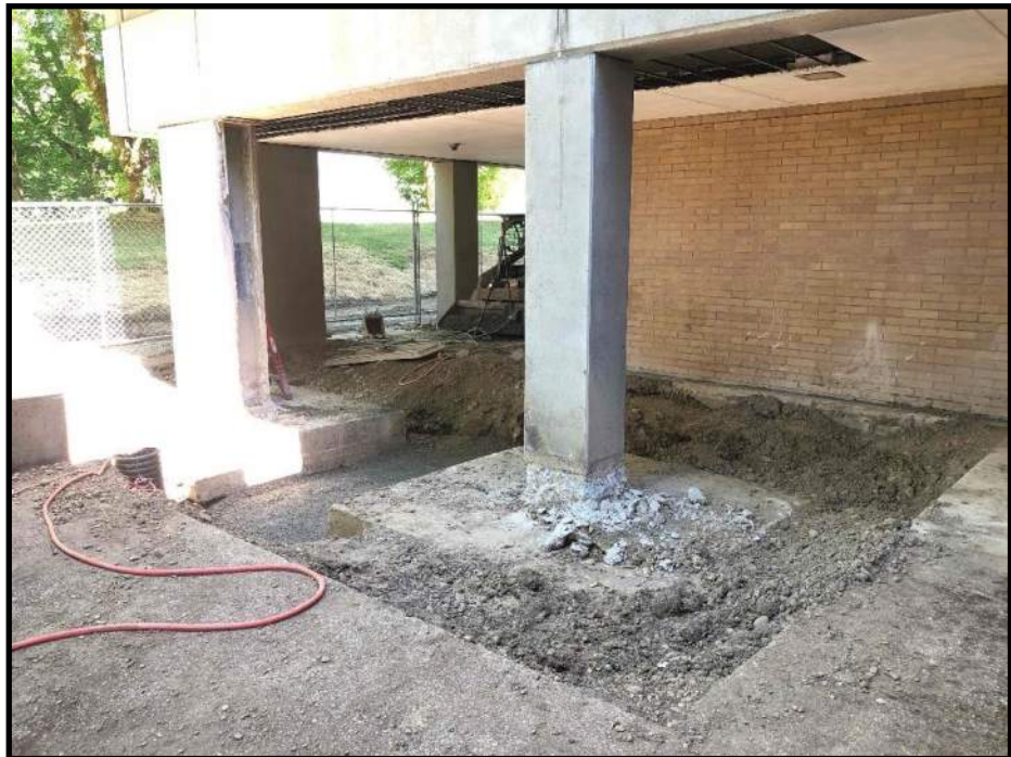
CVHS – Building A Seismic – SW shearwall footing excavations
