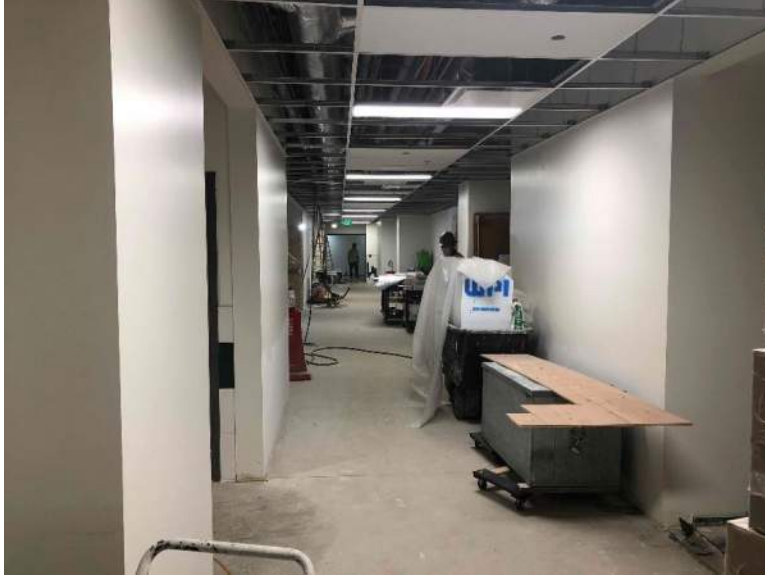
GES – North south hallway between area B-C
