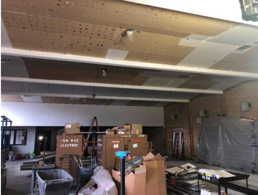
CMS Library ceiling ready for new acoustical glue on tile
