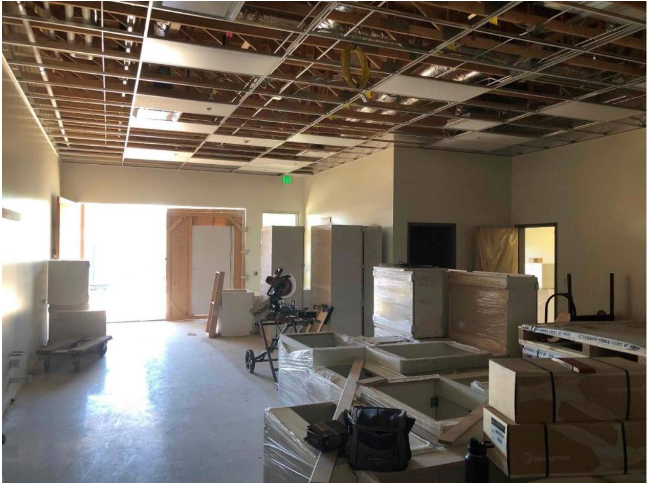
Area C – Art/Science Classroom progress
