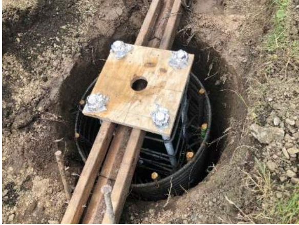
CHS – Covered Walkway – piles ready to place
