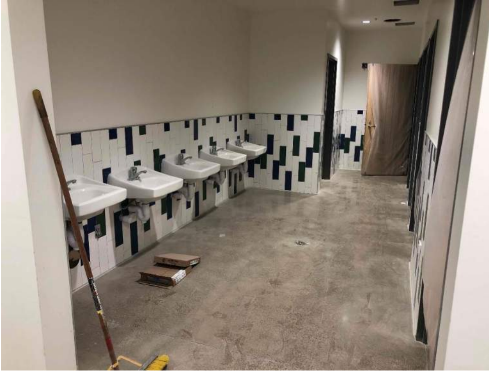
GES – Restroom progress
