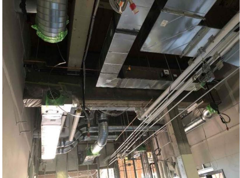
CVHS Building F – Ceiling rough-in HVAC & others near welding
