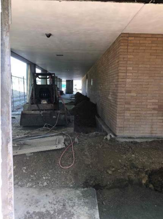
CVHS – Building A Seismic – West side footing improvements
