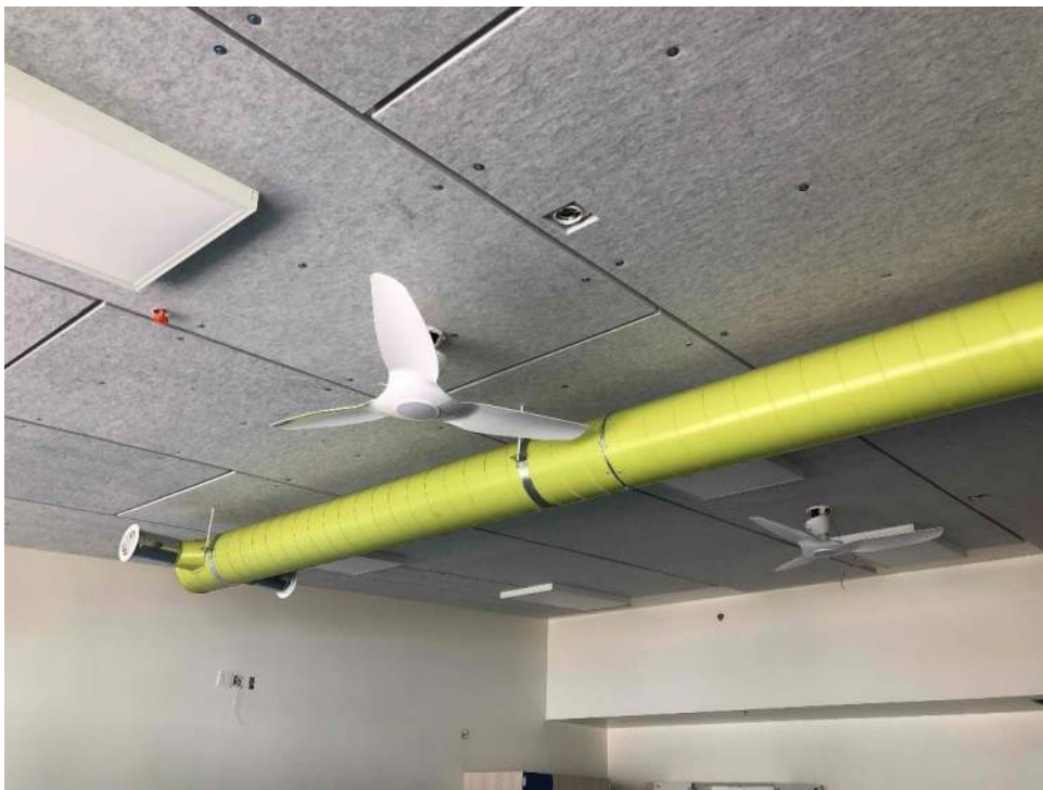
GES – Area C new classroom acoustical ceiling and partially painted ductwork
