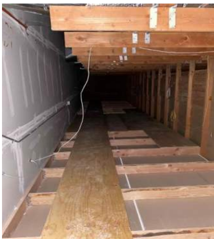
CMS – new soffit catwalk for future access
