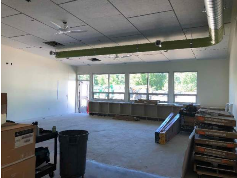
Garfield – Area C new classroom casework installing
