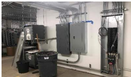
CVHS Building F – Electrical Room Progress
