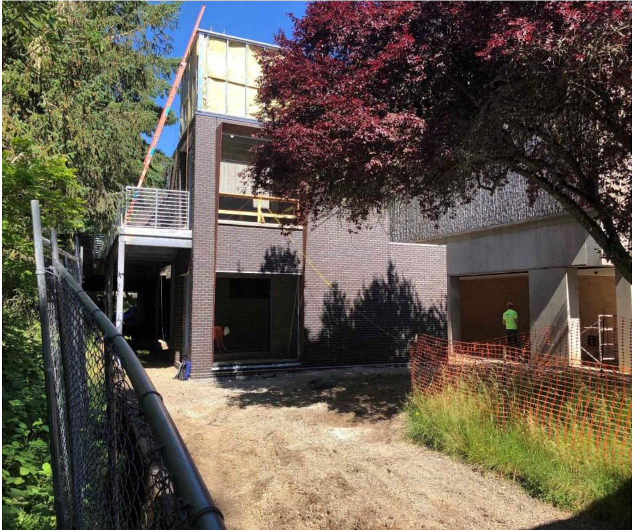
CVHS – Building A Elevator elevation view
