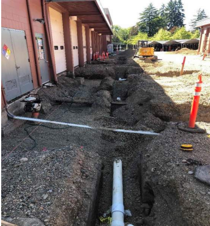
CHS – Covered work area utility installations
