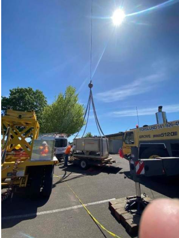
Crane picking HVAC unit to serve library
