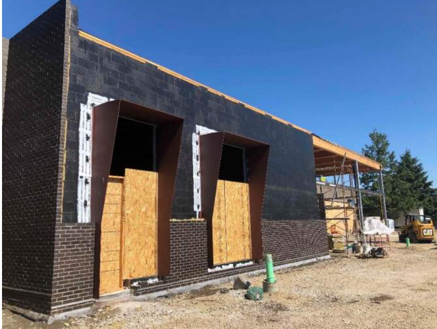
CVHS Building F – Exterior of new woods area
