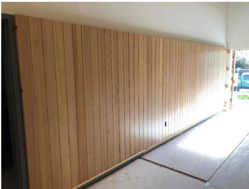
GES – North Gym Wall – reinstalled refurbished wood
