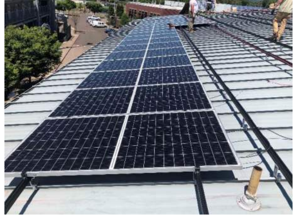
CHS- Solar expansion at east array
