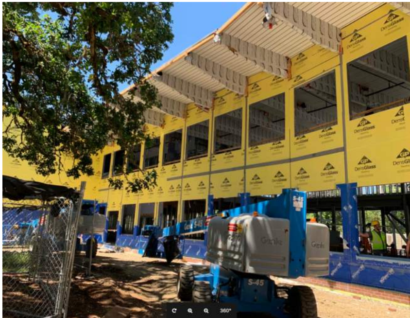
Exterior View of the commons
