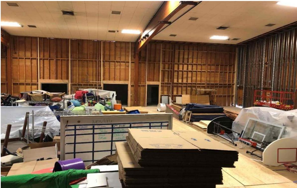
*Gym strongback wall work on right and new openings for PE office and storage*
