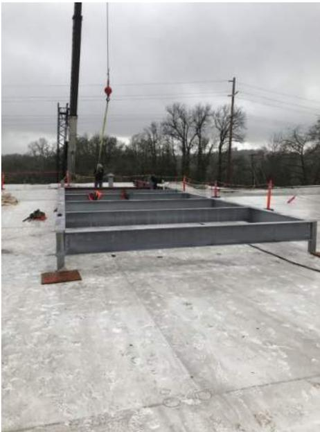
*CVHS – HVAC Roof support steel going in through holes in roof deck*
