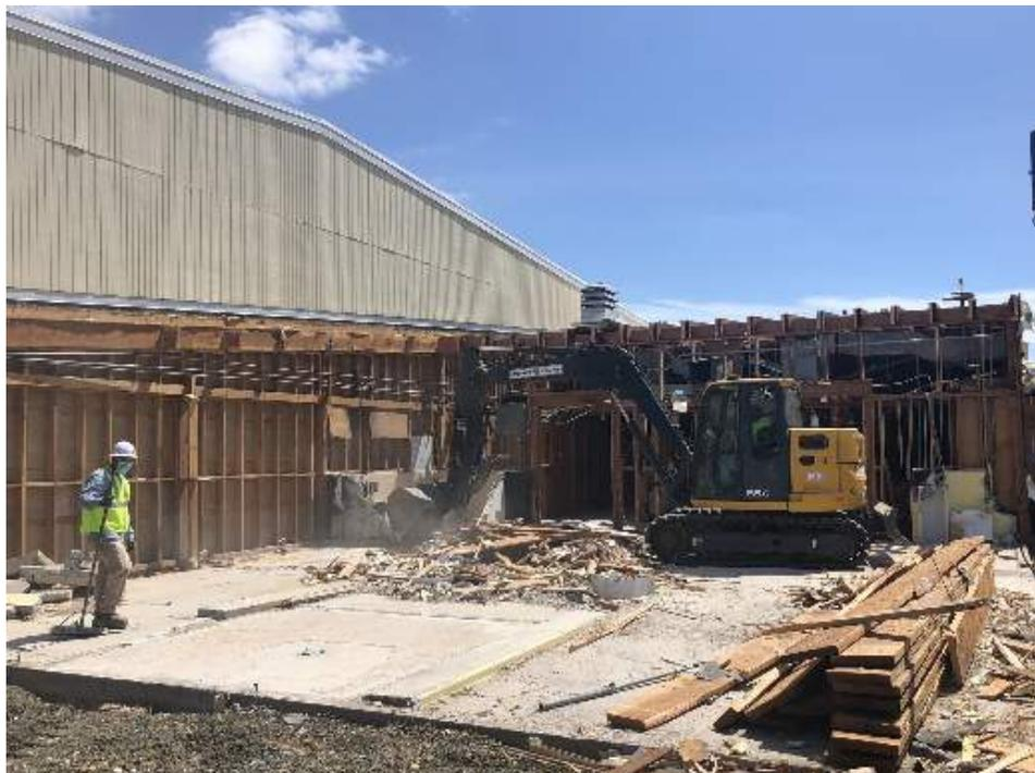
Old restroom and locker room area being demolished to make way for the new addition construction
