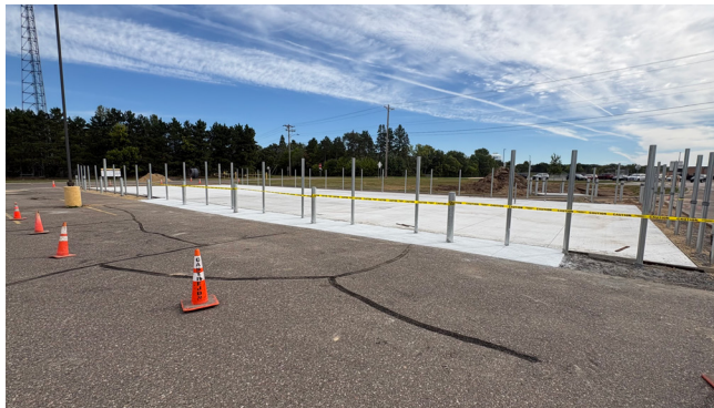
The site for the Elk River High School construction class's Habitat for Humanity home takes shape in the school's parking lot.
