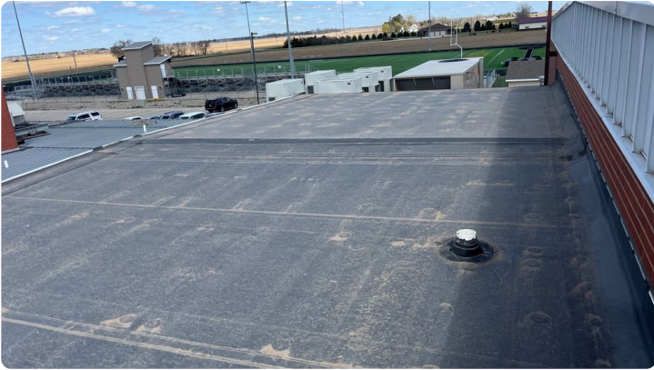
Photo showing overview Area 14 roof.
