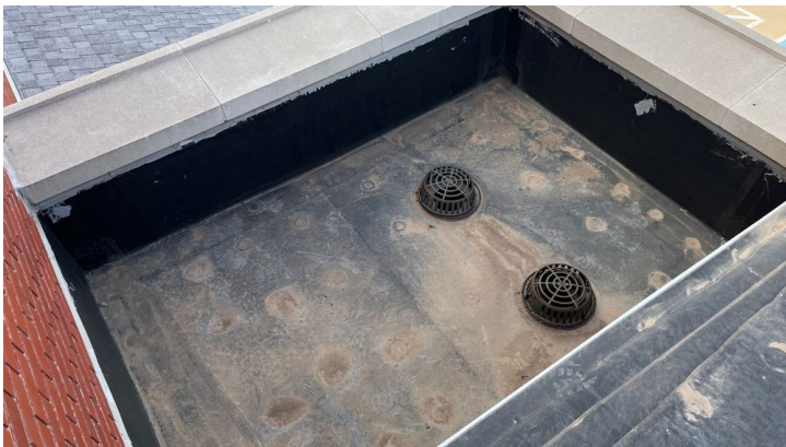
Photo showing additional overview of Area 05 roof.
