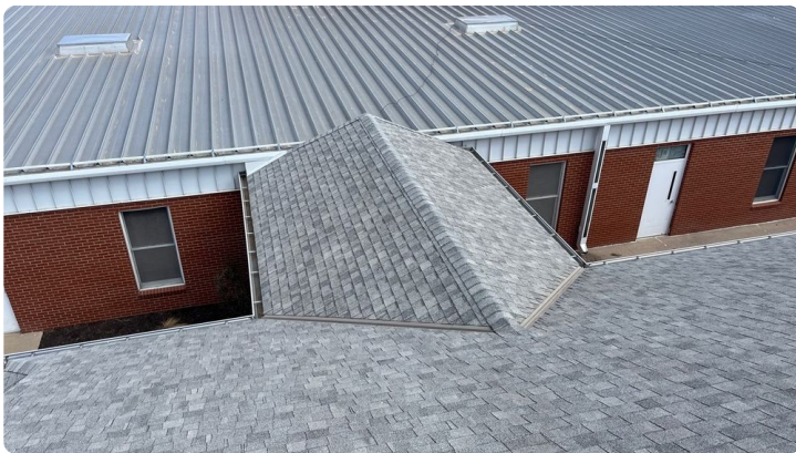
Photo showing additional overview of area 07 roof.
