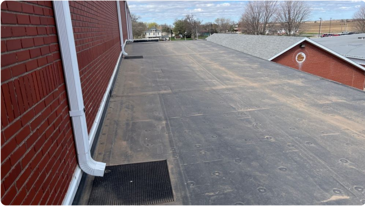
Photo showing overview of Area 04 roof.
