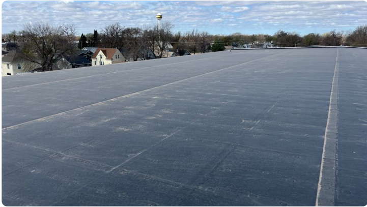
Photo showing overview of Area 02 roof.
