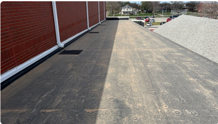
Photo showing additional overview of Area 04 roof.
