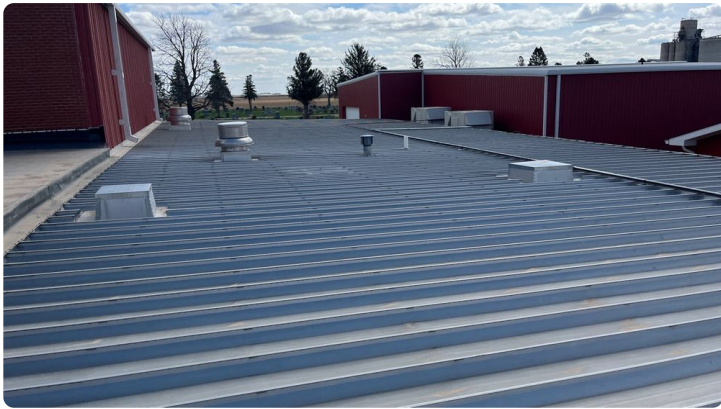
Photo showing additional overview of Area 13 roof.
