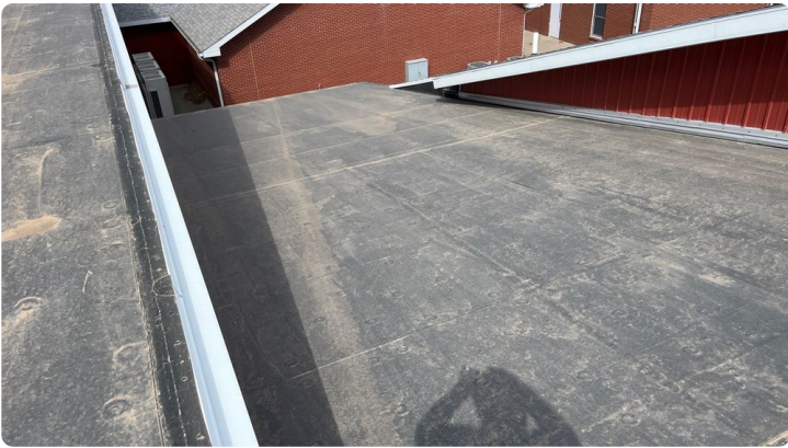
Photo showing additional overview of Area 04 roof.
