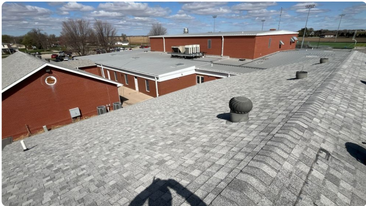
Photo showing additional overview of Area 03 roof.
