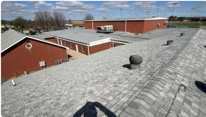
Photo showing additional overview of Area 03 roof.
