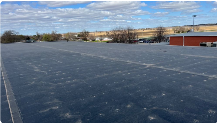
Photo showing additional overview of Area 02 roof.
