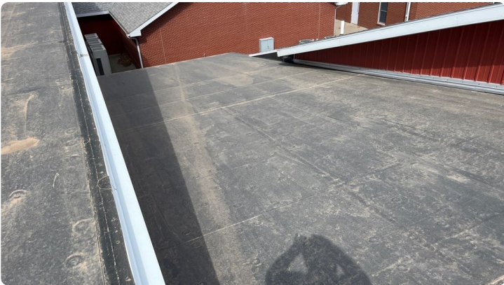
Photo showing additional overview of Area 04 roof.
