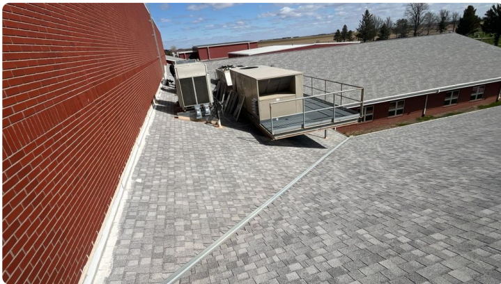
Photo showing additional overview of Area 01 roof.
