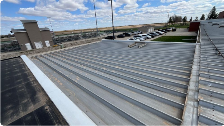
Photo showing overview of Area 11 roof.
