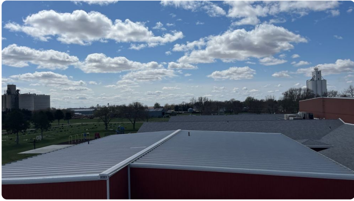
Photo showing overview of Area 17 roof.
