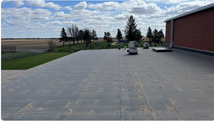
Photo showing overview of Area 12 roof.
