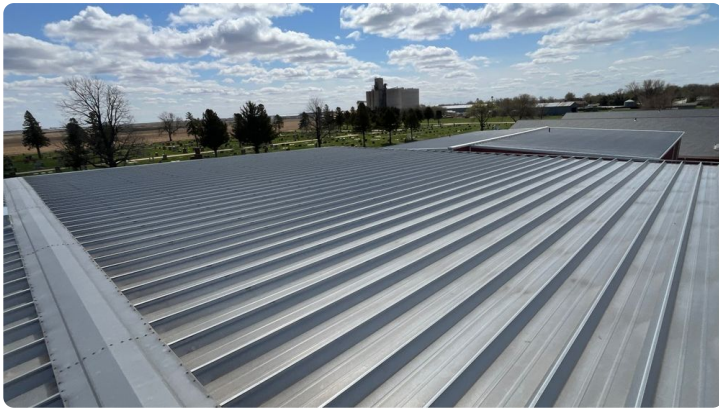
Photo showing overview of Area 15 roof.
