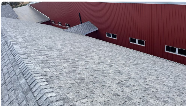
Photo showing additional overview of Area 07 roof.
