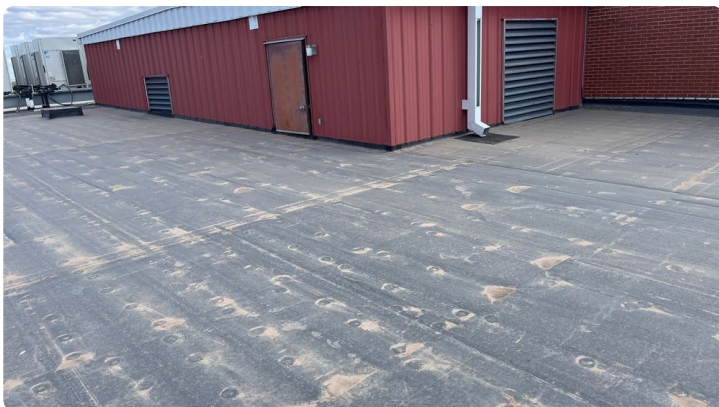
Photo showing additional overview of Area 12 roof.
