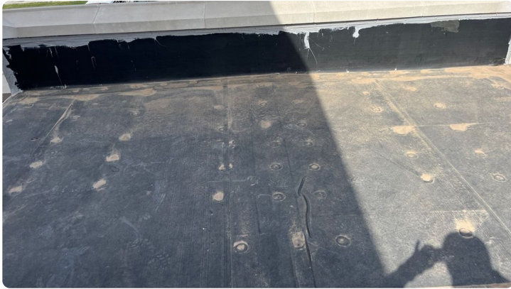
Photo showing overview of Area 05 roof.
