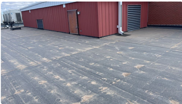
Photo showing additional overview of Area 12 roof.
