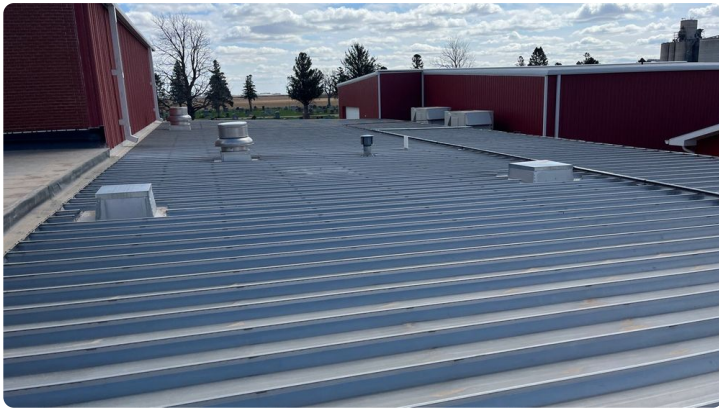
Photo showing additional overview of Area 13 roof.
