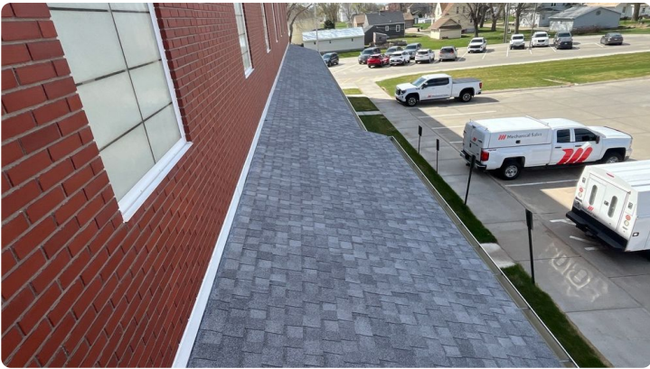
Photo showing overview of Area 06 roof.
