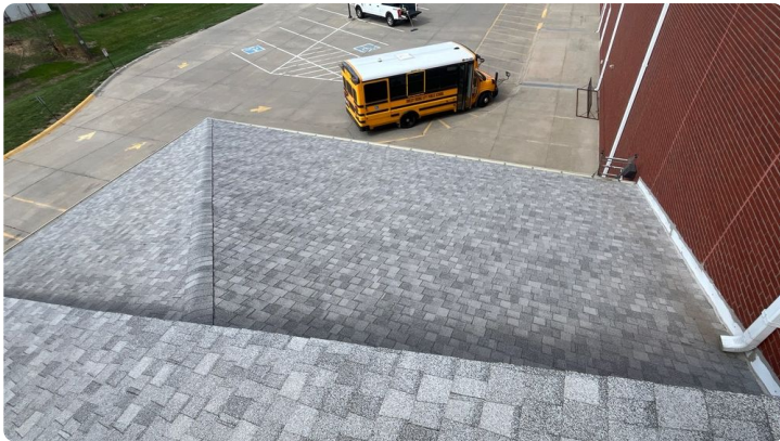
Photo showing additional overview of Area 01 roof.
