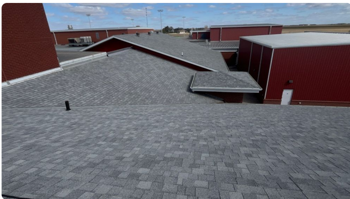
Photo showing additional overview of Area 01 roof.
