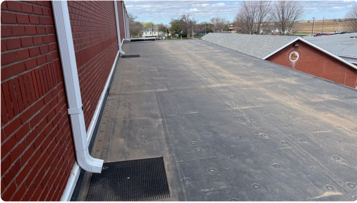
Photo showing overview of Area 04 roof.
