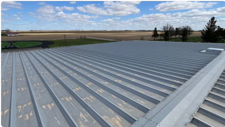
Photo showing additional overview of Area 15 roof.
