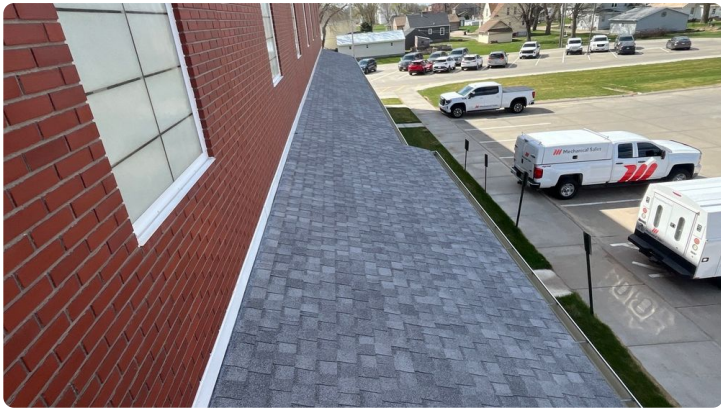
Photo showing overview of Area 06 roof.
