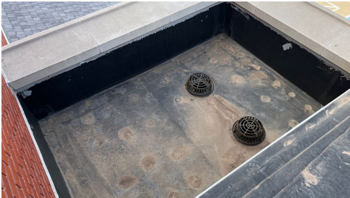
Photo showing additional overview of Area 05 roof.
