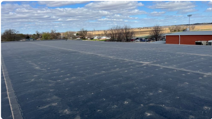
Photo showing additional overview of Area 02 roof.
