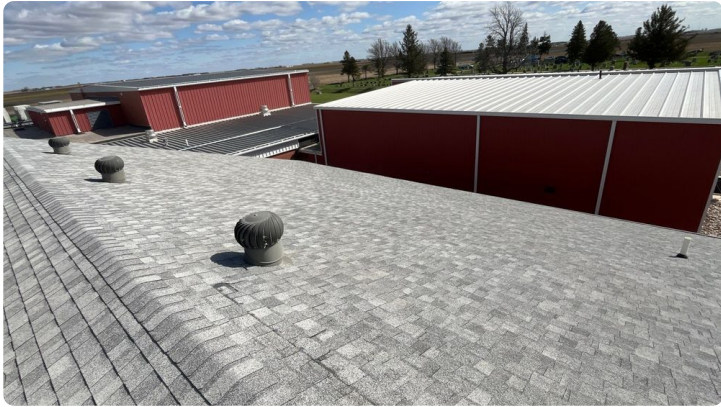
Photo showing overview of Area 03 roof.
