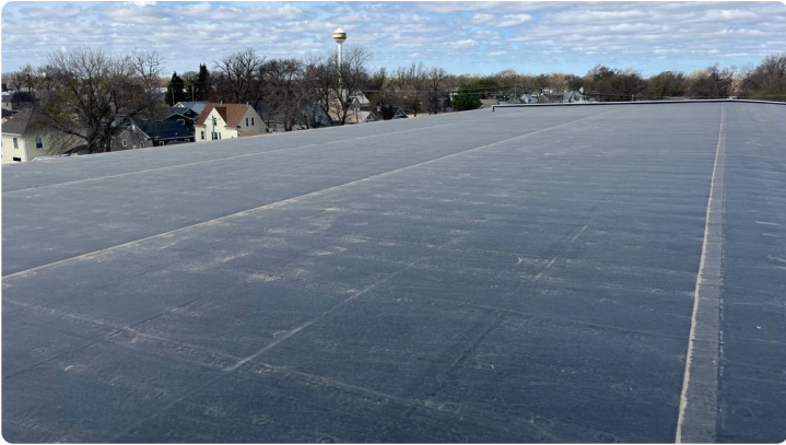
Photo showing overview of Area 02 roof.
