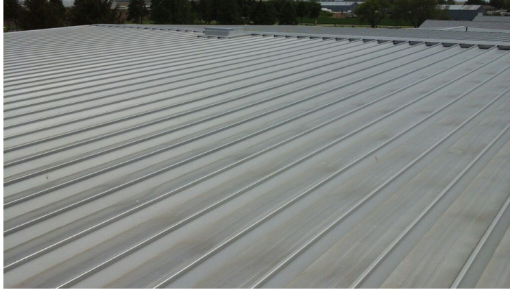
Photo showing overview of Area 15 Roof.
