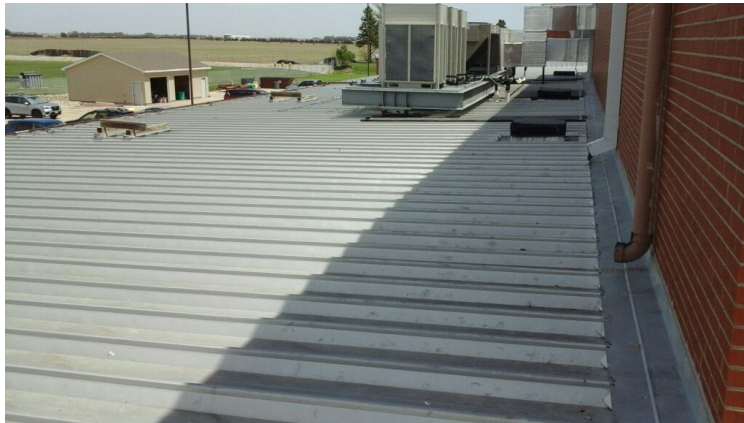
Photo showing additional overview of Area 09 Roof.
