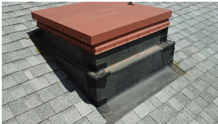
Photo showing rubber roof hatch projection.
