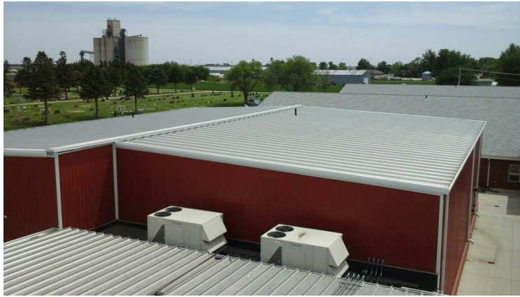
Photo showing overview of Area 17 Roof.
