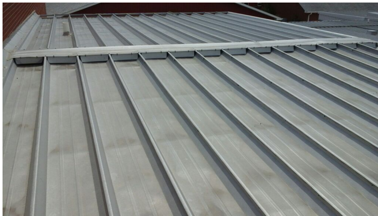
Photo showing overview of Area 14 Roof.
