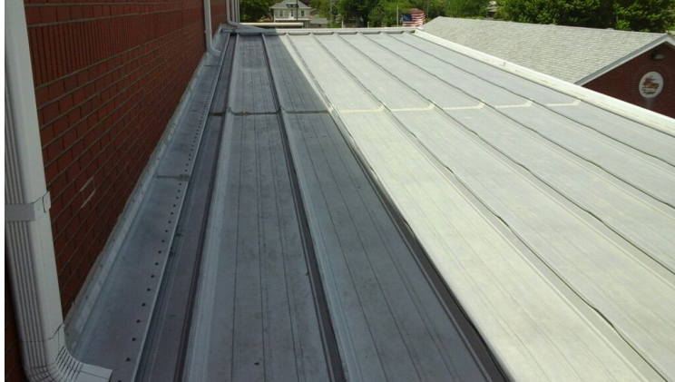
Photo showing overview of Area 04 Roof.
