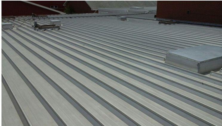
Photo showing overview of Area 13 Roof.
