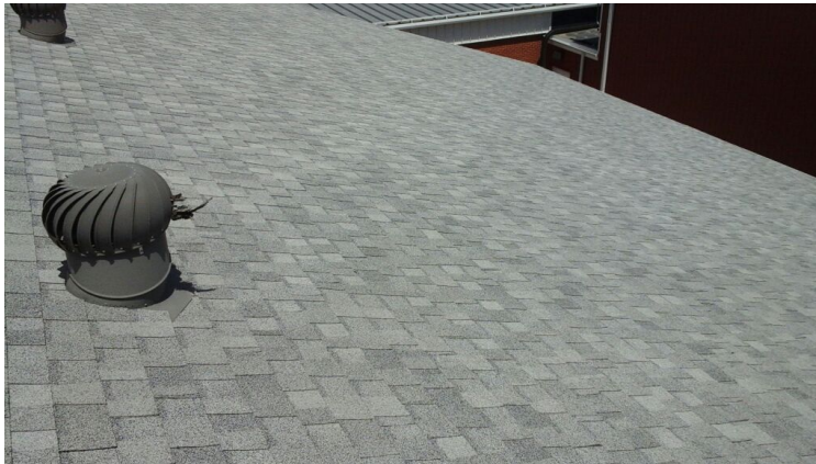
Photo showing additional overview of Area 03 Roof.
