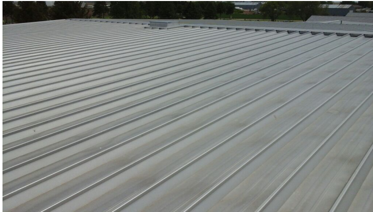
Photo showing overview of Area 15 Roof.
