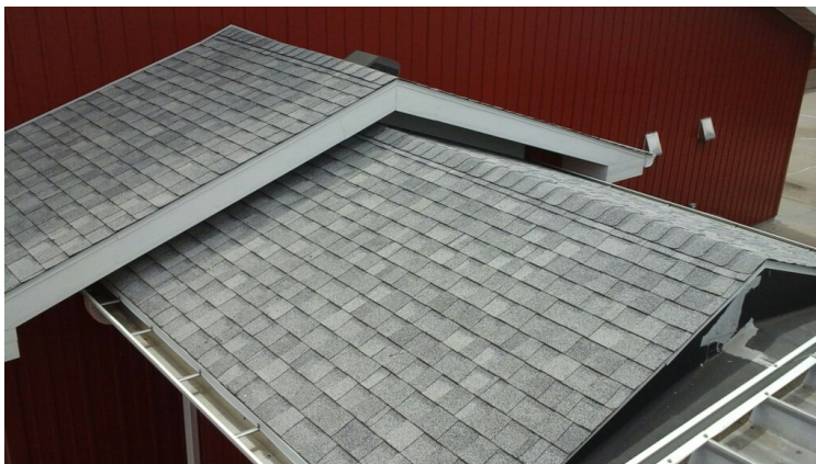
Photo showing overview of small adjacent shingled roof.
