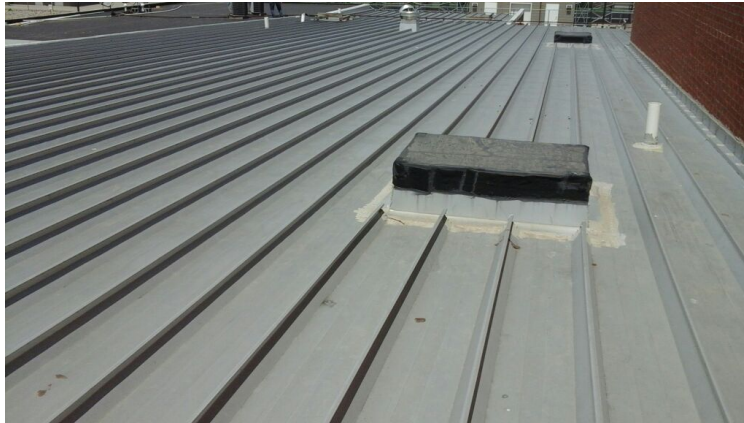
Photo showing overview of Area 09 Roof.
