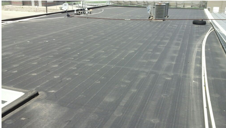
Photo showing overview of Area 10 Roof.
