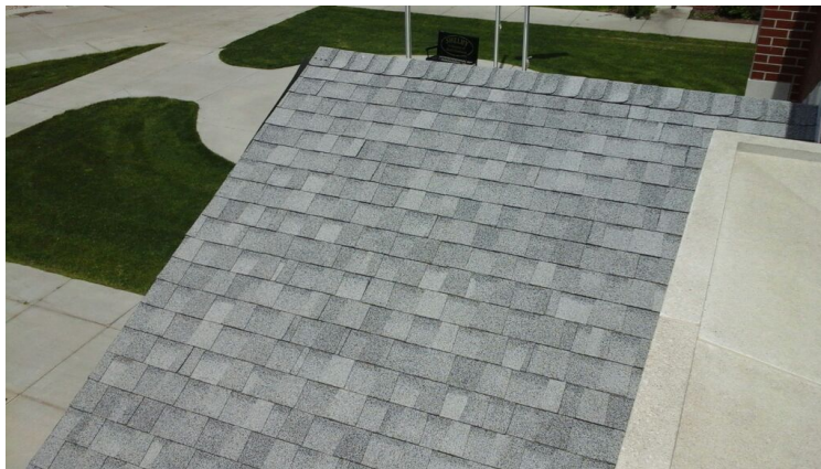
Photo showing additional overview of Area 06 Roof.
