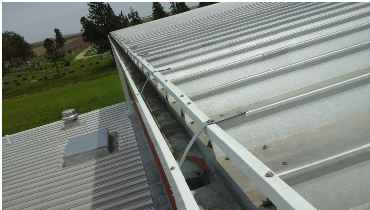
Photo showing condition of the gutter edge. Gutter is flush with metal roof which could cause issues with overflow.
