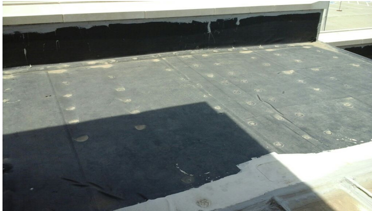
Photo showing overview of Area 05 Roof.
