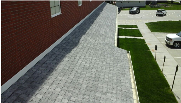
Photo showing overview of Area 06 Roof.
