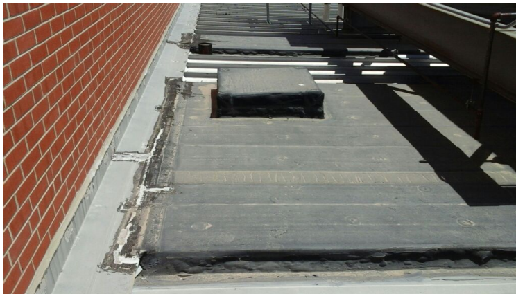
Photo showing future filled retrofit above HVAC units.
