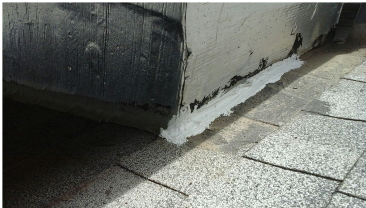
Photo showing temporary repair made where ineffective caulking was pulled up.
