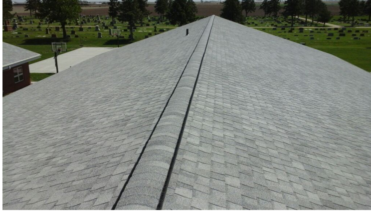
Photo showing overview of Area 01 Roof.
