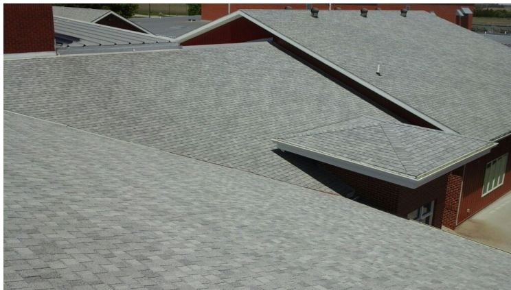
Photo showing additional overview of Area 01 Roof.
