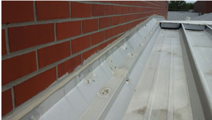
Photo showing condition of the perimeter flashings.
