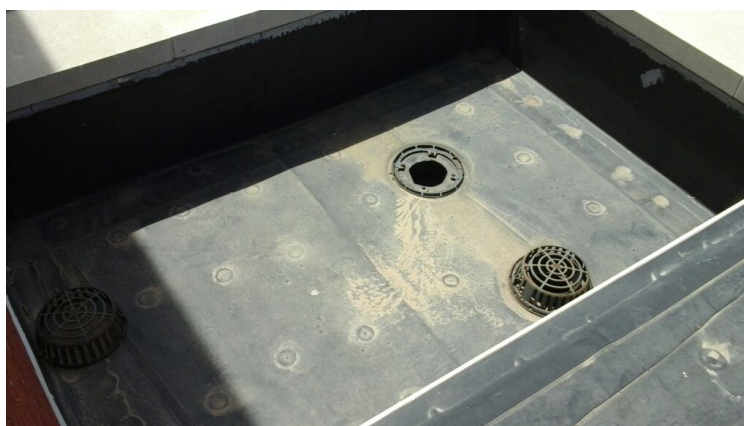
Photo showing additional overview of Area 04 Roof.
