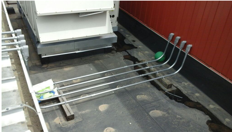
Photo showing overview of small adjacent rubber roof.
