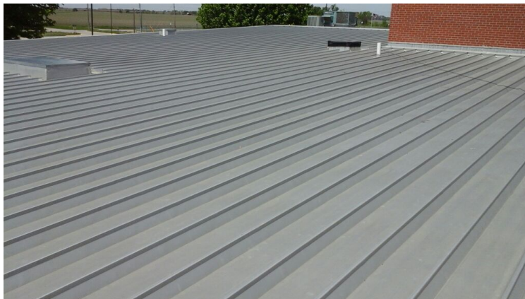
Photo showing additional overview of Area 08 Roof.
