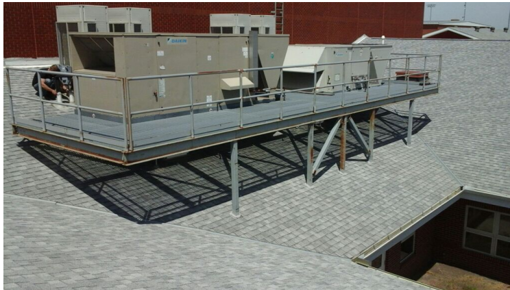
Photo showing additional overview of Area 01 Roof.
