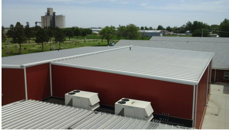
Photo showing overview of Area 17 Roof.
