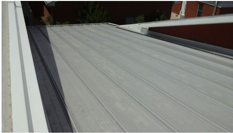
Photo showing additional overview of Area 04 Roof.
