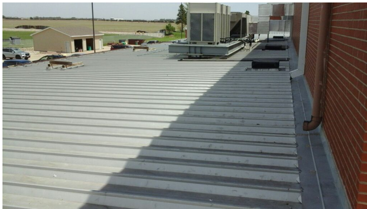
Photo showing additional overview of Area 09 Roof.
