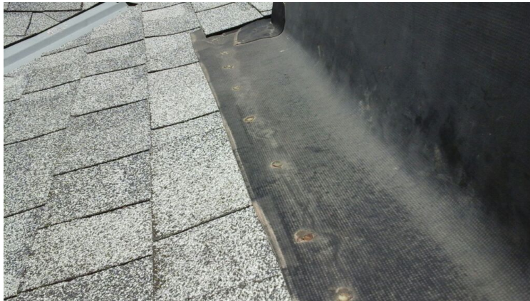
Photo showing nails through rubber into shingles below.
