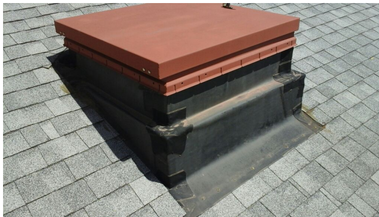
Photo showing rubber roof hatch projection.
