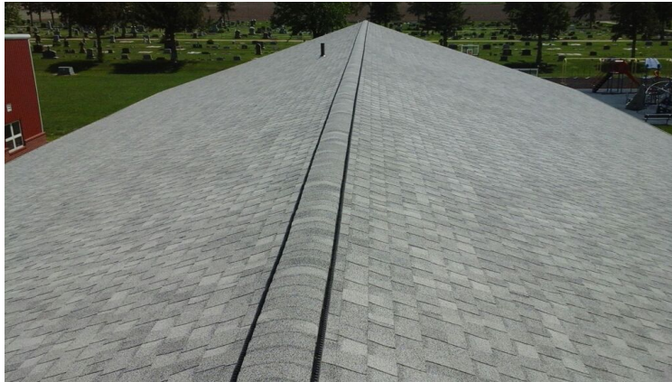
Photo showing additional overview of Area 01 Roof.
