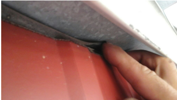
Photo showing area under gutter where rubber does not fully flash wall. Exposed framing underneath.
