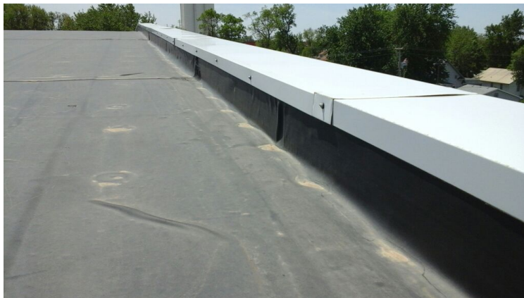
Photo showing condition of the perimeter flashings.
