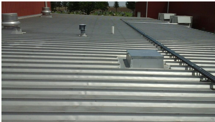
Photo showing additional overview of Area 13 Roof.
