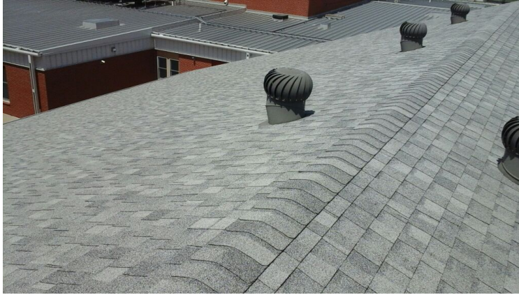
Photo showing overview of Area 03 Roof.
