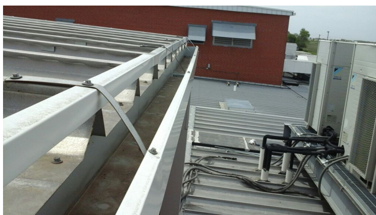
Photo showing condition of the gutter edge. Top of gutter is even with metal roof. Potential back flow issue into area directly below that is exposed.
