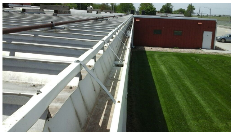
Photo showing condition of the gutter edge. This gutter is appropriately attached with top lower than metal roof.
