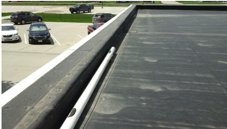
Photo showing condition of the perimeter flashings.
