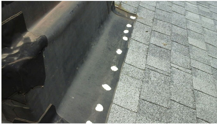
Photo showing temporary repair made to the nail penetrations in rubber.
