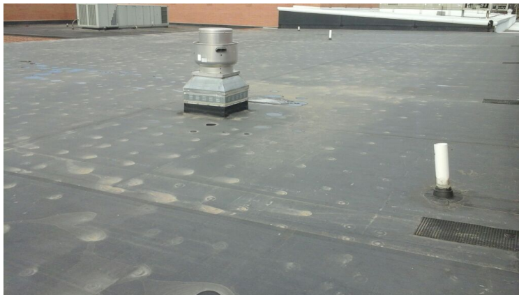
Photo showing overview of Area 04 Roof.
