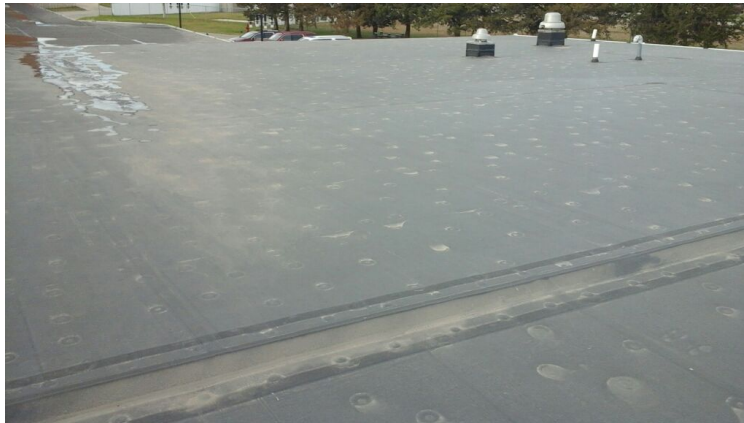
Photo showing additional overview of Area 09 Roof.
