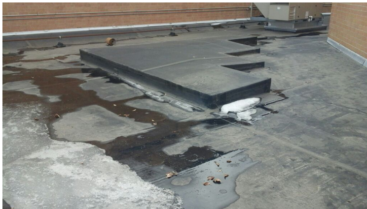
Photo showing additional overview of Area 13 Roof.
