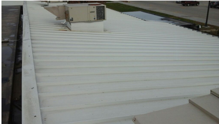
Photo showing overview of Area 10 Roof.
