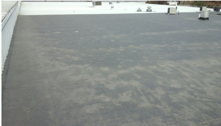
Photo showing overview of Area 09 Roof.
