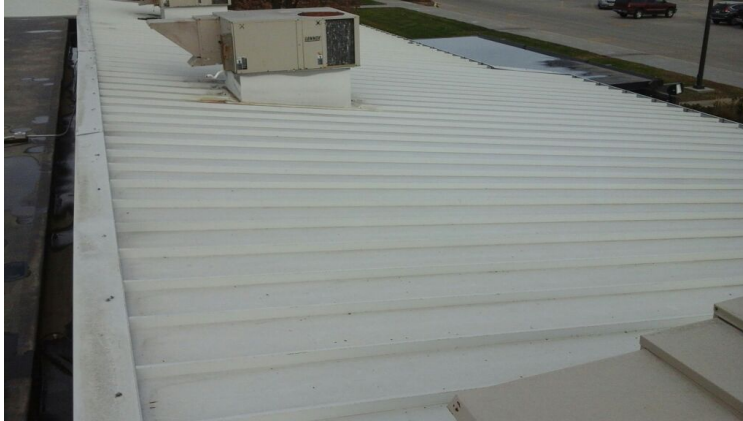
Photo showing overview of Area 10 Roof.
