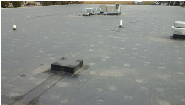
Photo showing additional overview of Area 09 Roof.
