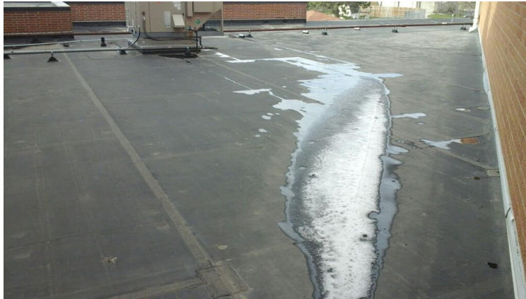
Photo showing additional overview of Area 13 Roof.
