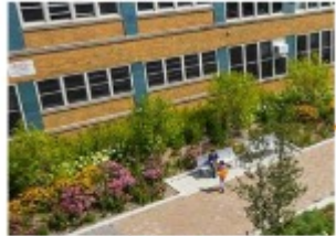
Asphalt Removal & Landscaping
