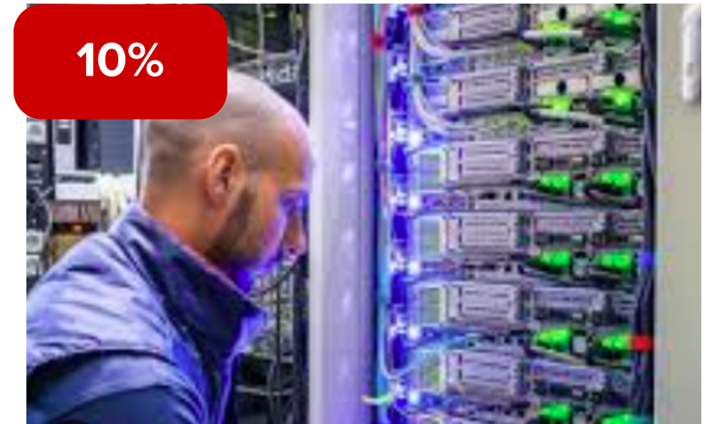
Storage & Backup Updates
