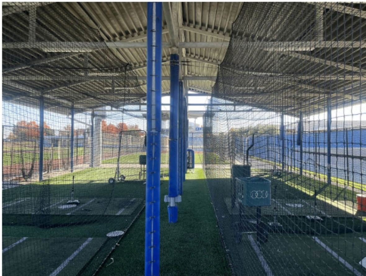
Midlothian High School Batting Tunnels
