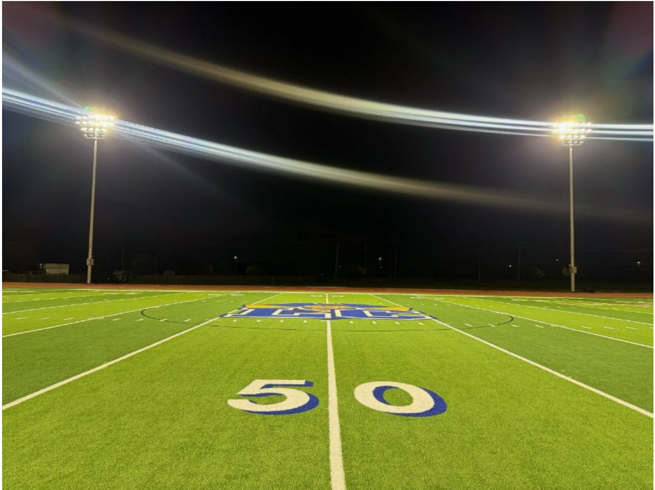
Lakeview HS – New Lighting
