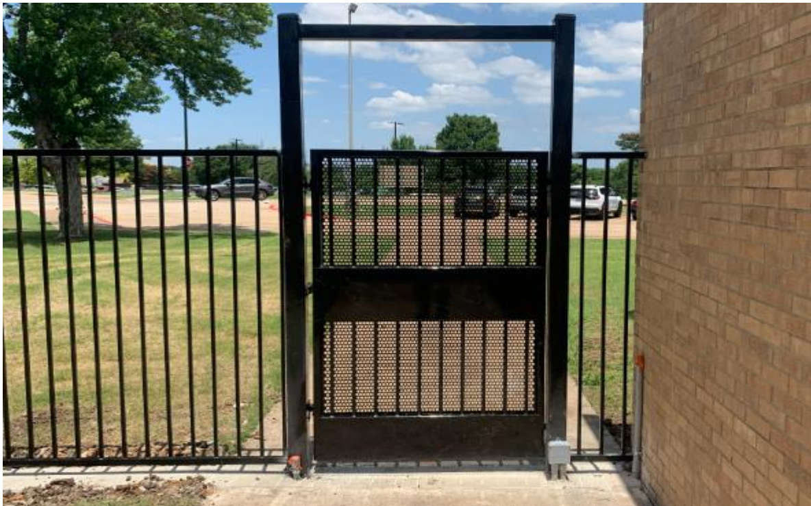
Pedestrian Gate limits access at Spring Creek ES
