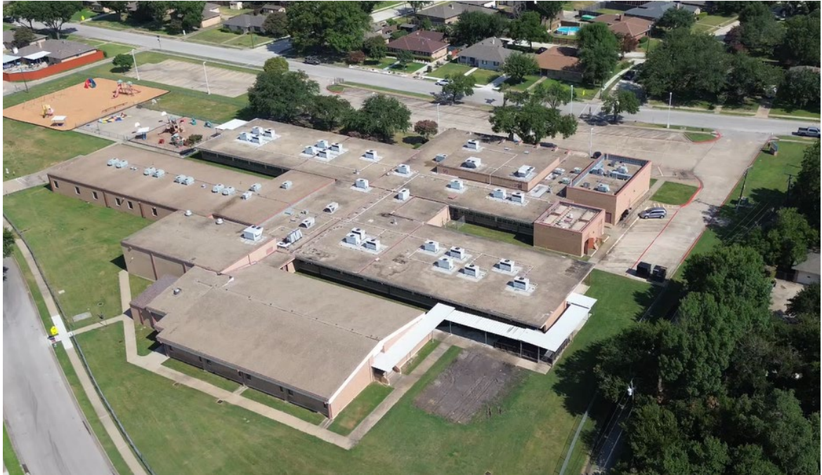
Paragon Roofing and LBL are working with GISD Maintenance to make sure roof-top units are disconnected and removed safely and remain intact.
