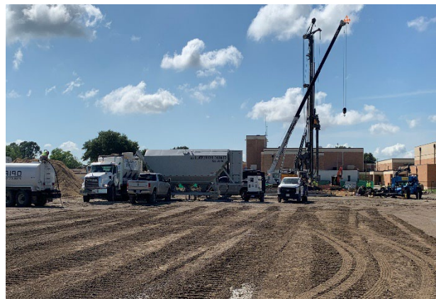
South Garland: Progress
