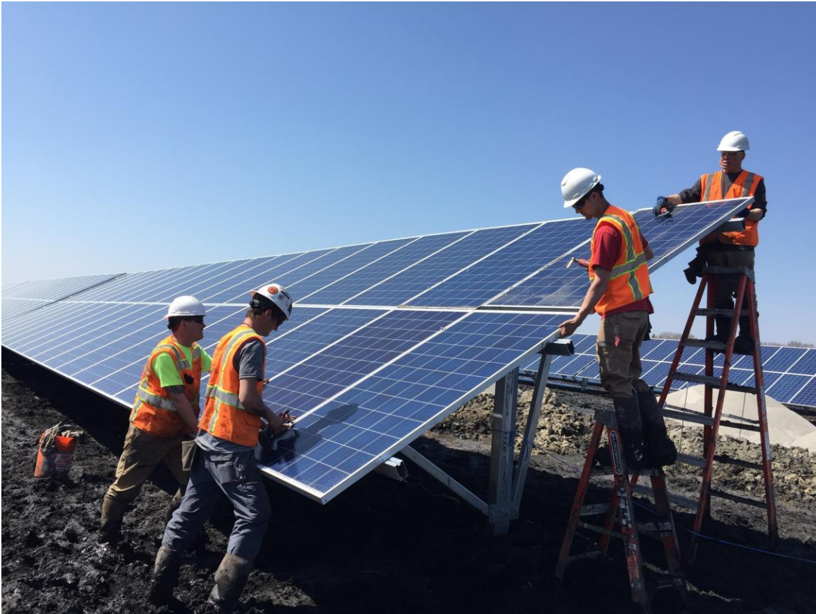
NES crew construction one of our 1 MW AC Community Solar projects
