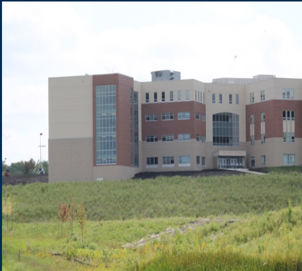
New Classroom Wing
