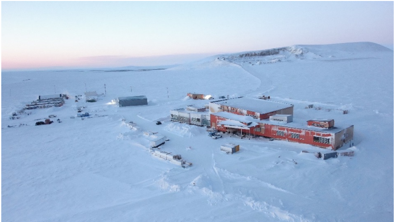
Aerial of the Replacement Kivalina School taken early January 2022
