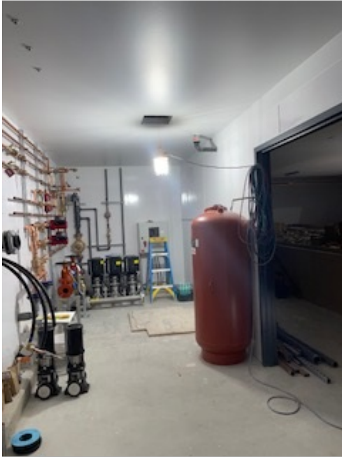
WWTF interior progress
