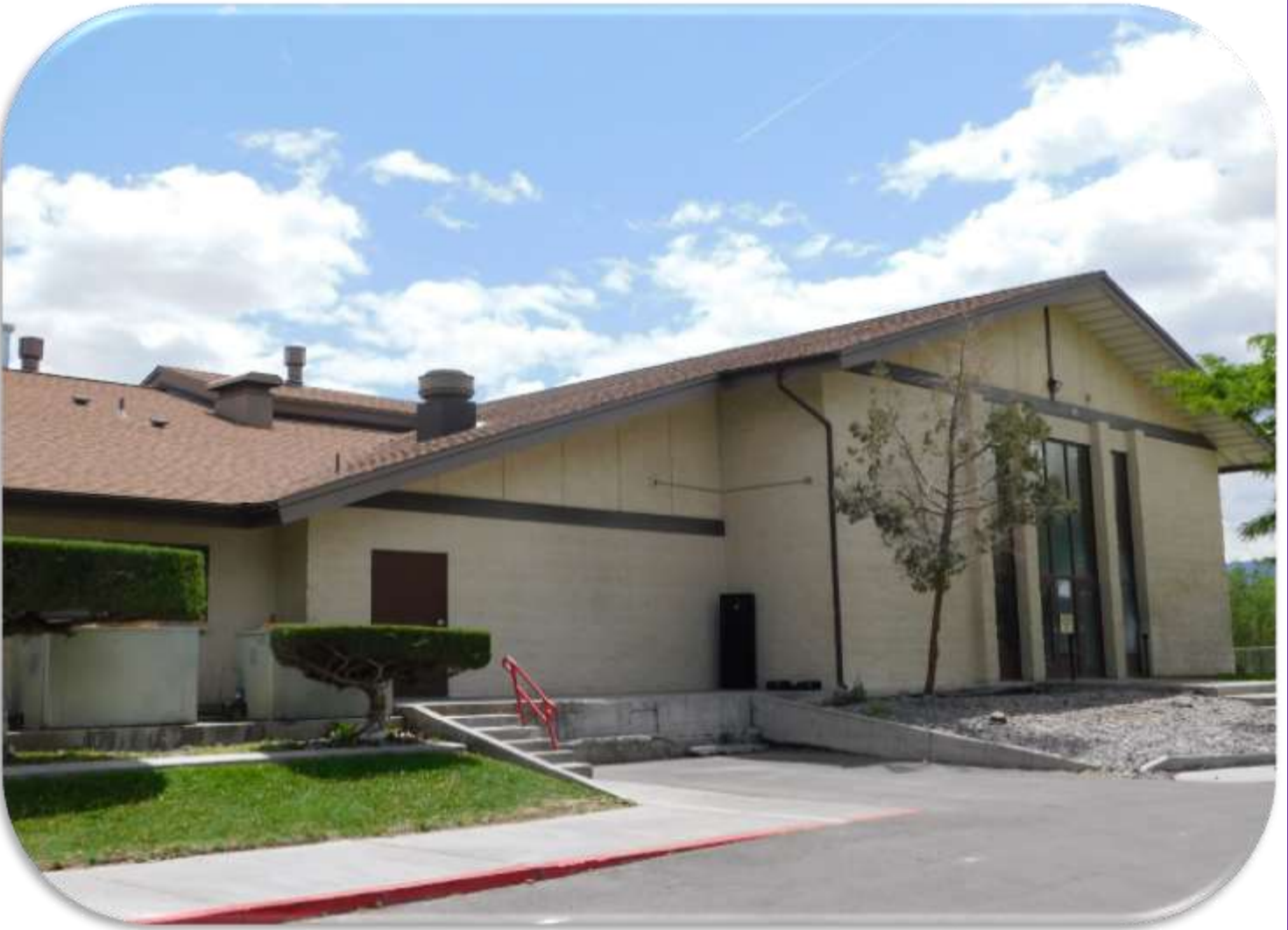
(FIS) STREET VIEW OF THE BUILDING TO BE RE-ROOFED.
