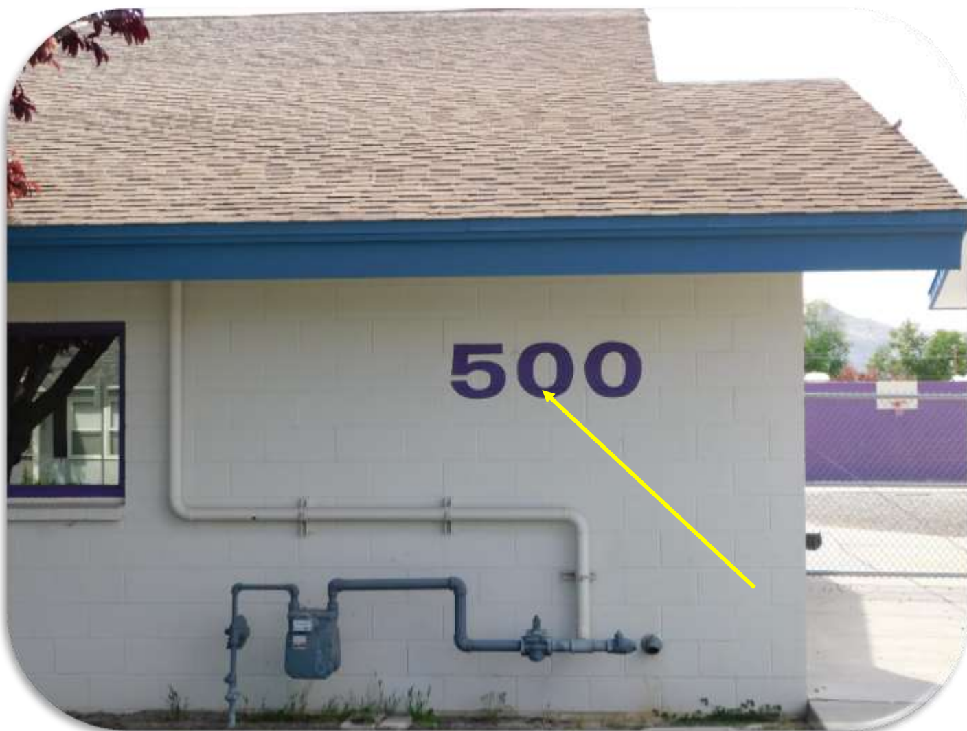
BUILDING 500 AT YERINGTON ELEMENTARY.
