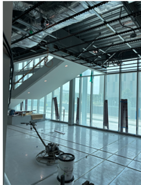
Level 1 – West Lobby Terrazzo Install
