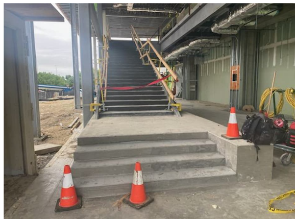
West Lobby – Monumental Stair
