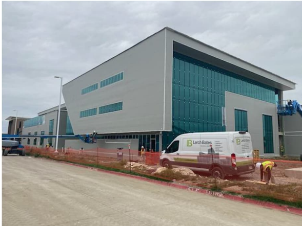
East Elevation – Glazing nearing completion
