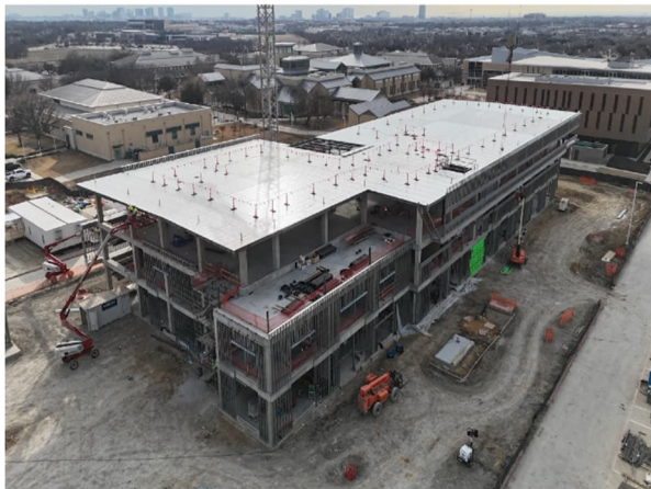
Southwest Corner of Building
