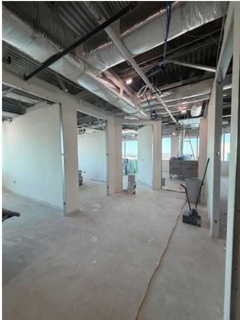
4 th Floor – Phase 3 New Offices
