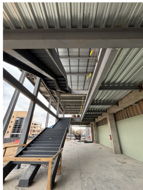
West Monumental Stairwell
