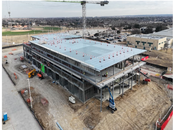
Northwest Corner of Building
