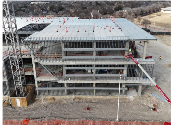
Southeast Corner of Building
