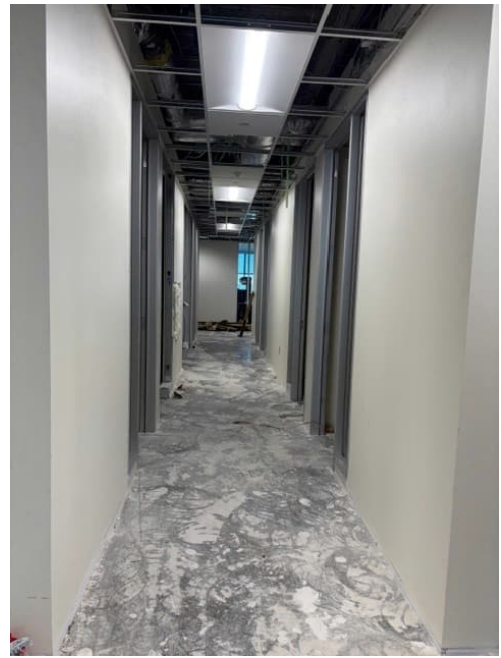
3 rd Floor – Phase 3 New Offices
