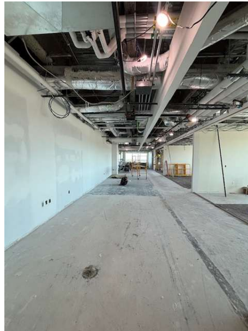
4 th floor – Presidential Suite Offices
