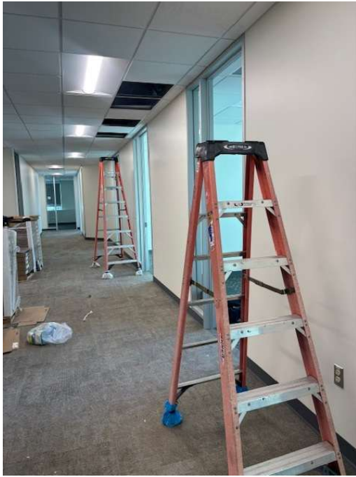
1 st Floor – New Foundation Offices
