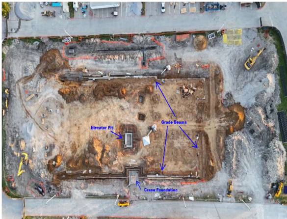
Overview highlighting grade beams, elevator pit and crane foundation
