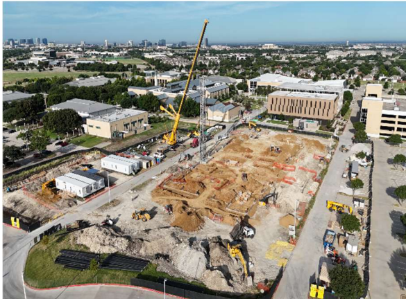
View to Southwest and partial crane install
