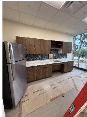
1st Floor – Staff Breakroom
