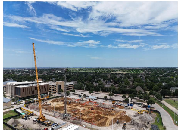
View to Northwest with crane fully installed
