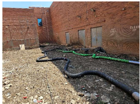
Fine Arts Courtyard Hydro Vac
