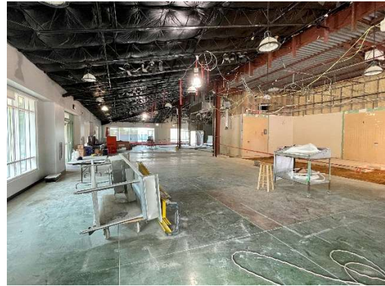
Interior Renovation in Dining Hall
