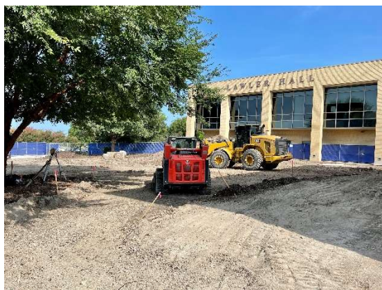
Prepping New Entrance Area for Lawler Hall
