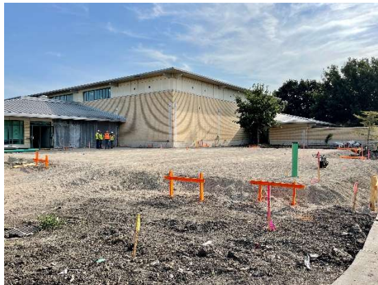
Building Pad for Kitchen Additions
