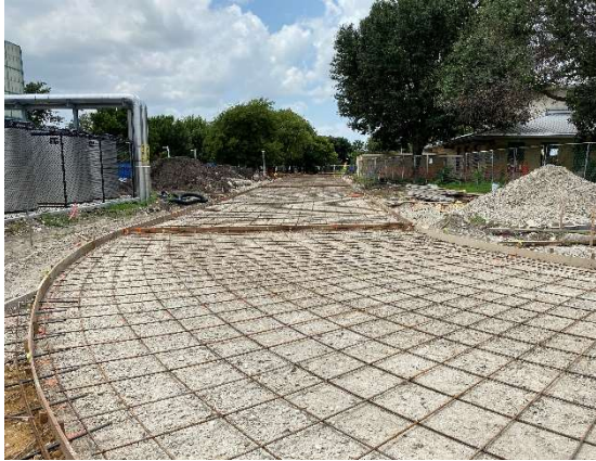
Form and Rebar for Fire Lane
