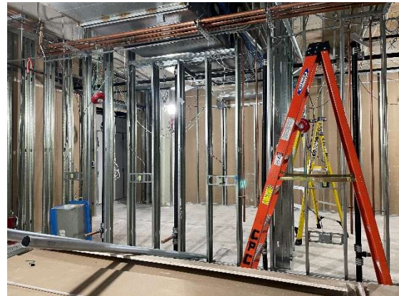
Framing in Dental Area Renovation
