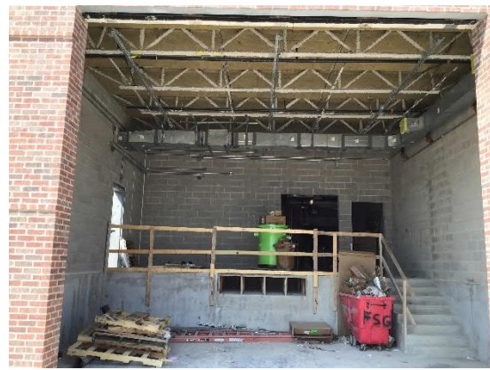
Loading Dock Area
