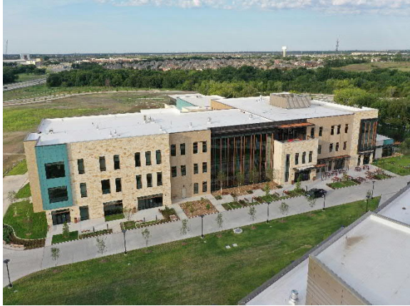
North View of Student Center
