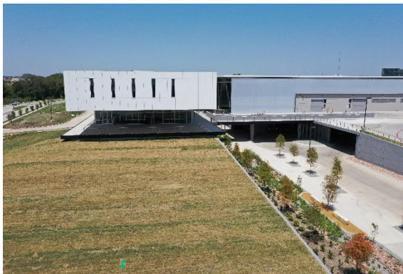
South View of Academic Building
