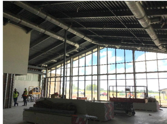
Curtain Wall at Library Area
