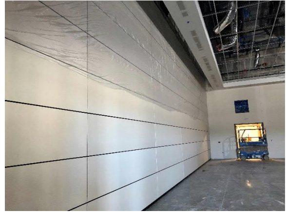
Partition Installed in Conference Center Room
