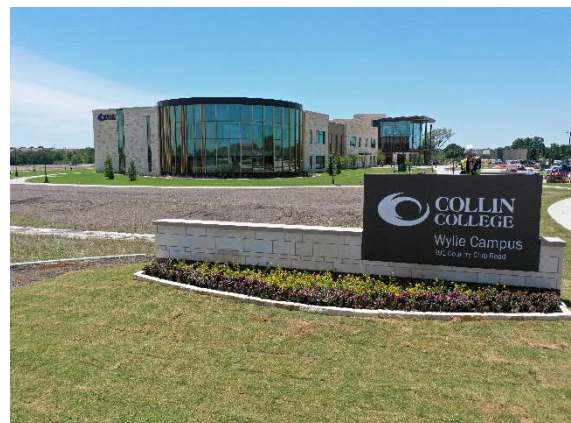
North Entrance Monument Signage
