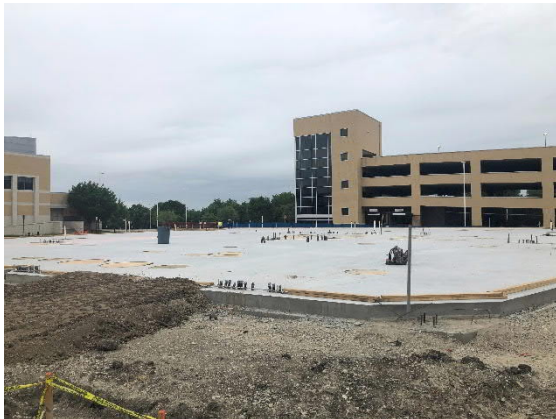
Concrete Poured in Area A
