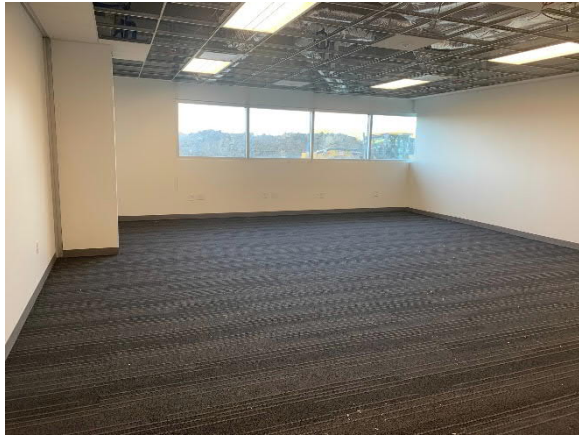
Carpet Installed in Mockup Class in Academic Building
