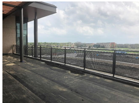
Terrace Railing Panels Installed at Library
