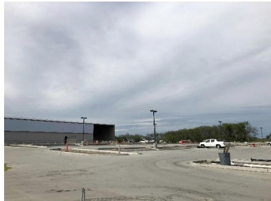
Light Poles Installed in South Parking Lot
