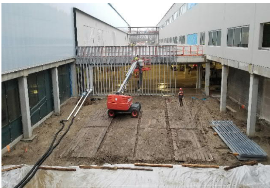
Five Star Installing Screen Wall
