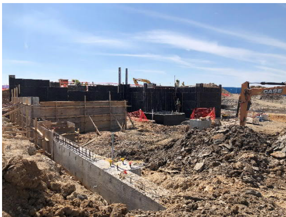
Grade Beams Forming for South Building
