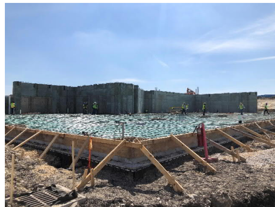
Walls Being Formed at North Building
