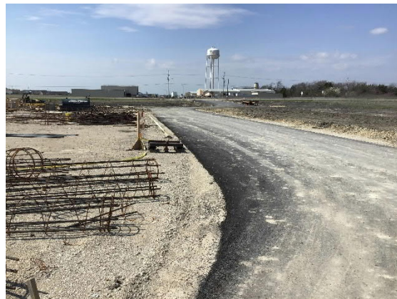
Site's North Fire Lane
