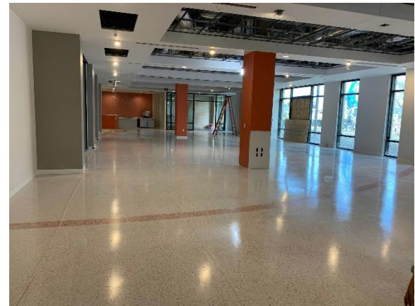
Terrazo Flooring at Student Dining Area
