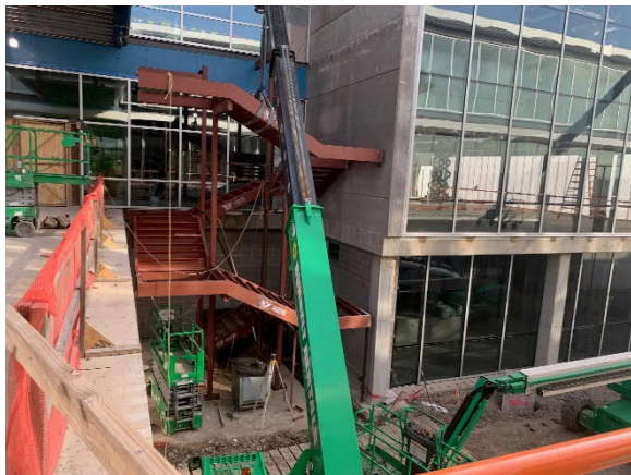
Stair Installation outside of Trade Bar B
