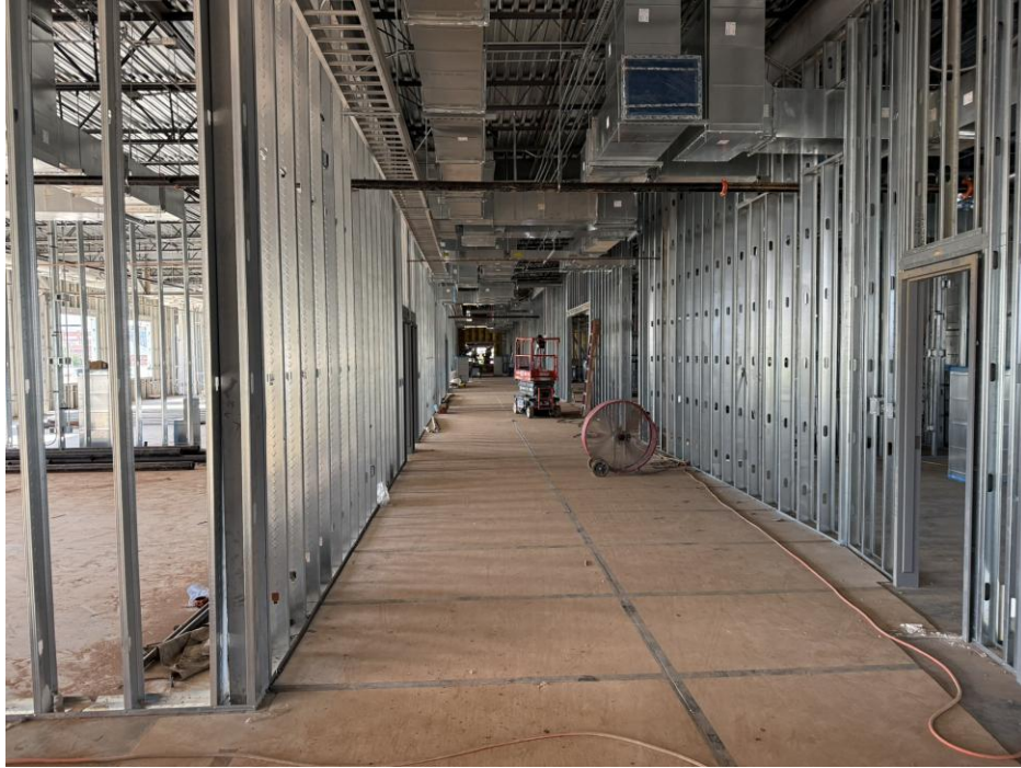
AREA 5 – SECOND FLOOR HALLWAY
