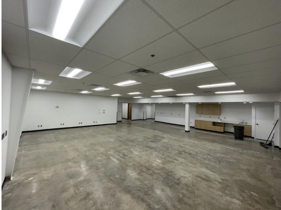
RENOVATED EXISTING BREAK / MEETING ROOM
