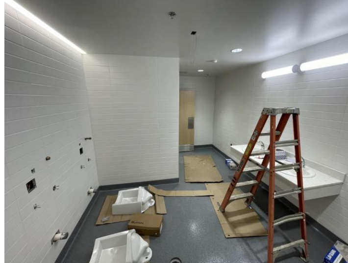
TRANSPORTATION BUS DRIVER RESTROOM
