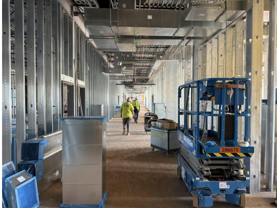
AREA 5 – SECOND FLOOR HALLWAY
