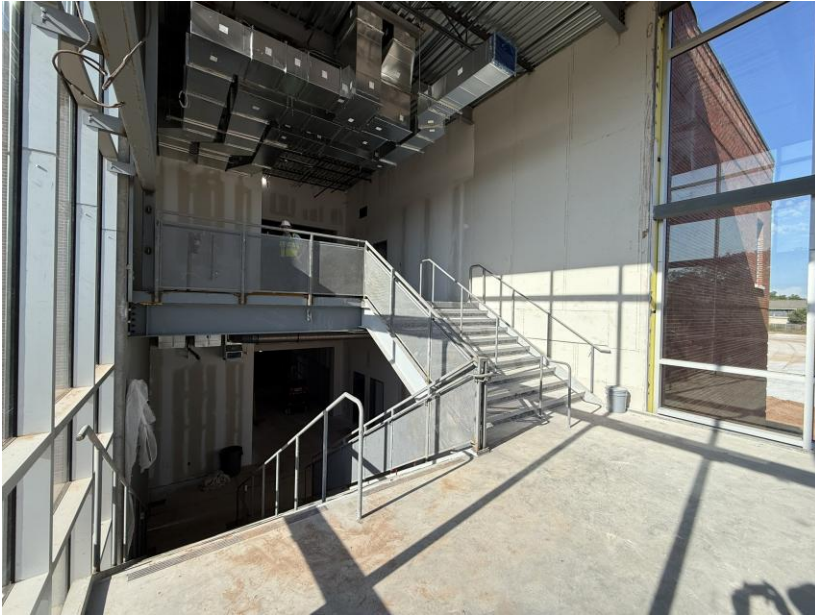
AREA 1 – NORTH STAIRS
