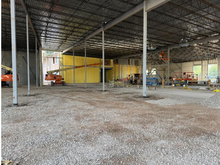
AREA 6 – PA WING STRUCTURAL FRAMING AND PRECAST WALLS
