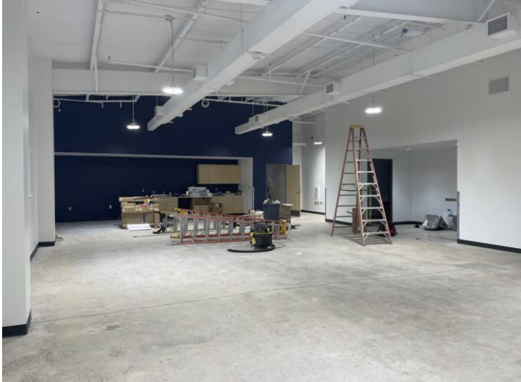
TRANSPORTATION BUS DRIVER BREAKROOM AREA
