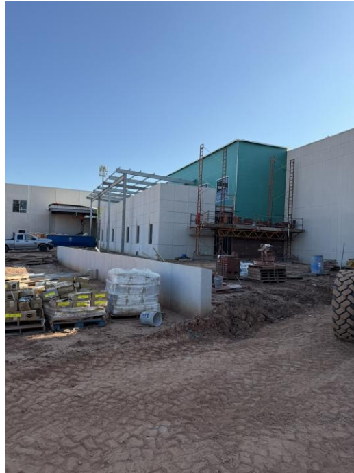
AREA 4 – WEST SIDE PATIO AREA
