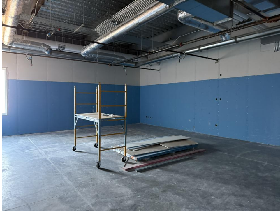
AREA 2 – SPED CLASSROOM (HIGH IMPACT GYPSUM BOARD)
