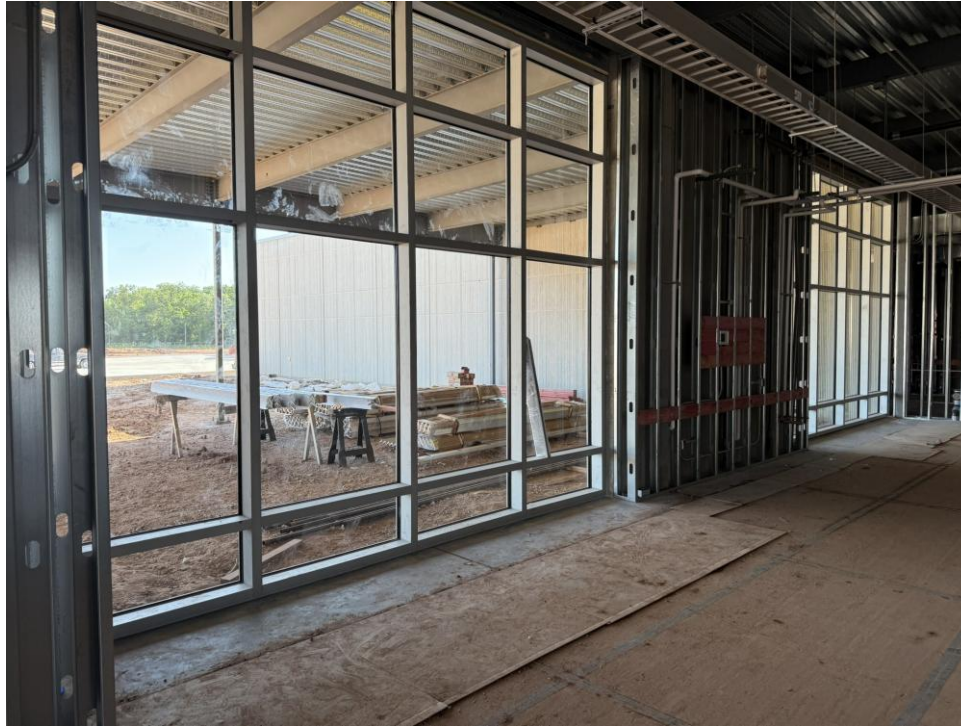
AREA 2 – SPED HALLWAY AT COURTYARD
