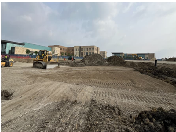
Building Pad Preparation
