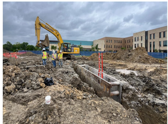
Trenching for Underground Utilities
