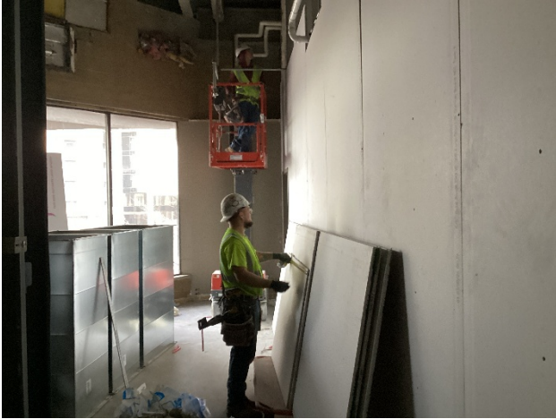
1st Floor Drywall Installation
