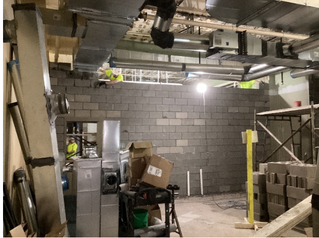
1st Floor CMU Walls
