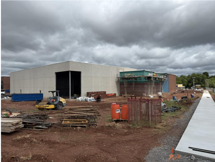
AREA 6 – PA WING SW EXTERIOR
