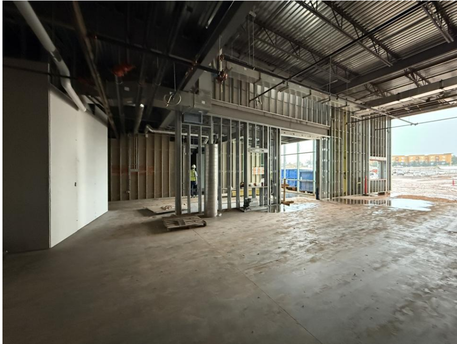
AREA 4 – RECEPTION / ENTRY LOBBY
