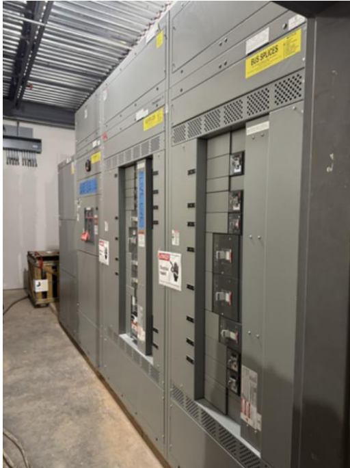
AREA 5 – ELECTRICAL ROOM BUILD OUT
