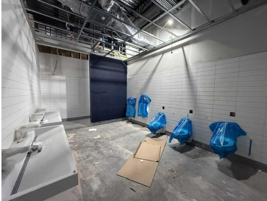
AREA 3 – BOYS RESTROOM
