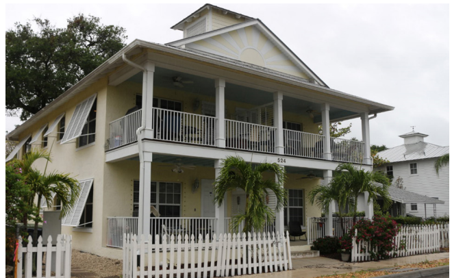
A 2-STORY PORCH ON AN APARTMENT BUILDING.
